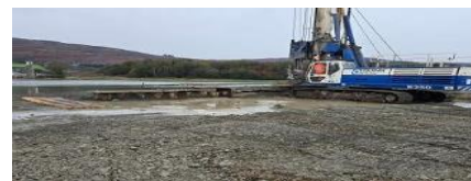
Piling Works Northern Embankment.
