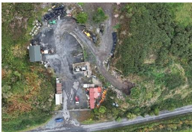
Drone Footage taken by the Facilities Team in October showing the site and boundary of the Bush Depot. Credit: Dean Hearty
