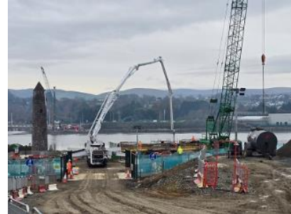
Concrete Pour Rear Wall Southern Abutment
