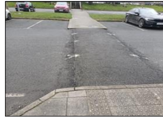
Resurfacing and repair works on ramps at Drogheda Aura Leisure Centre
