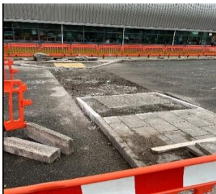
Repair works on ramps at Drogheda Aura Leisure Centre
