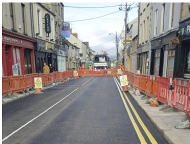
Phase A Completed
