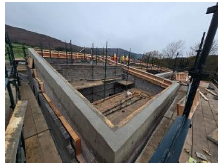
Ring Beam on Control Building
