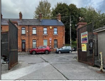
Current access to Fair Street Machinery Yard, off Greenlanes, Drogheda
