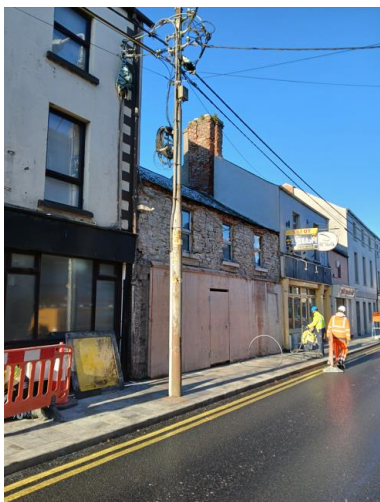
Phase A Completed
