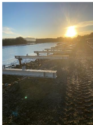
Substructure of Boardwalk being assembled
