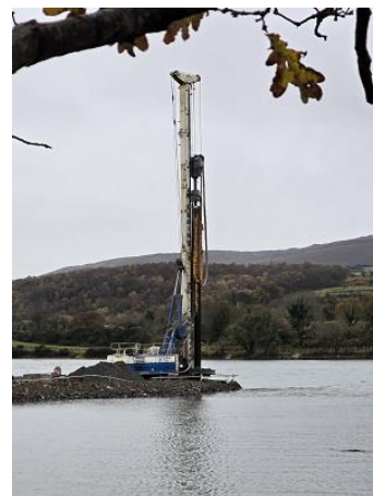
Piling Platform Northern Embankment
