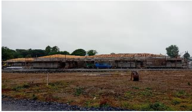
School Building under construction
