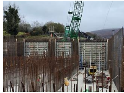
Shuttering and Steel Reinforcement Southern Abutment
