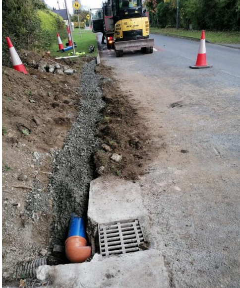
Drainage on the L-2318 Tullyallen
