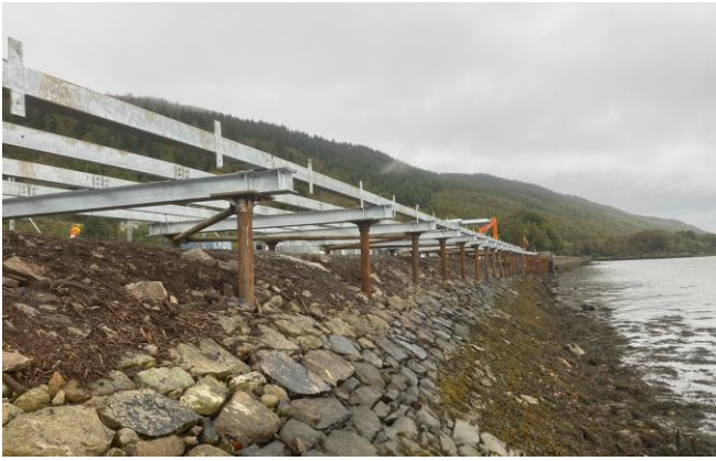
Substructure including Piles
