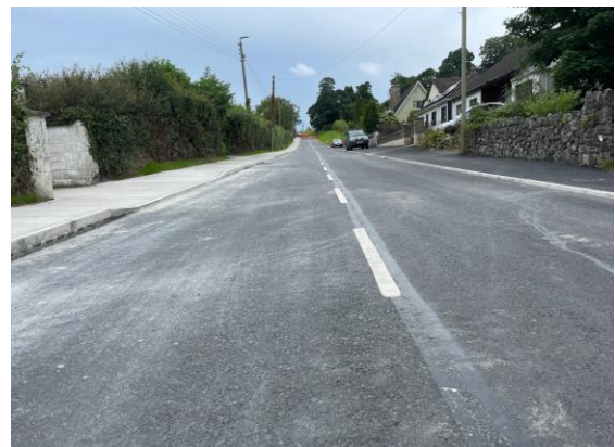
Basecourse at Castletown Rd Section.
