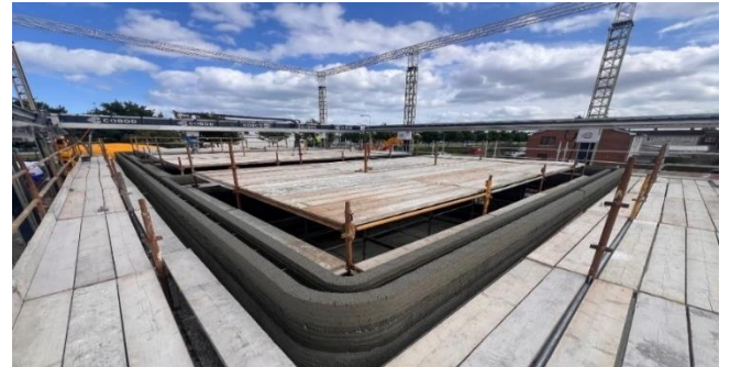
3D Concrete Printing Pilot Project at Grange Close, Dundalk
