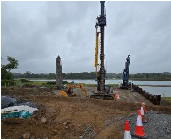
Installation of cofferdam southern embankment.
