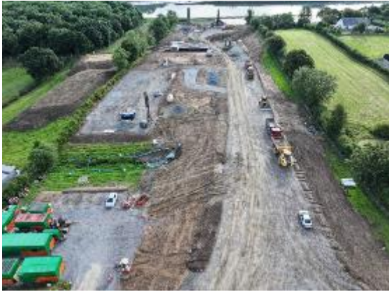
Roadworks Southern Approach.
