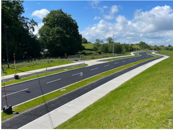
Section of carriageway nearing completion. Works south of Castletown Cross
