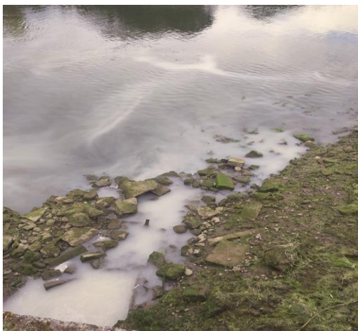
Sewage overflow discharging to Boyne
