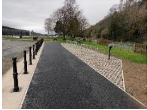
Works Complete in Victoria Lock in NI
