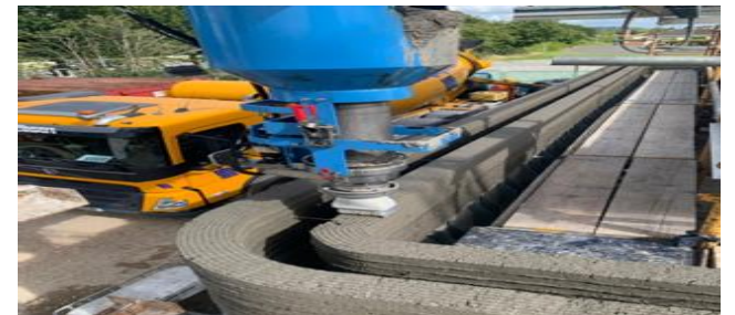
3D Concrete Printing Pilot Project at Grange Close, Dundalk
