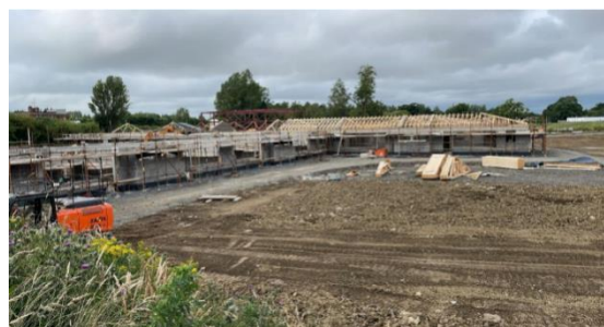
Overall site Progress
