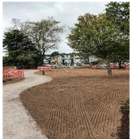
Landscaping Works nearing completion
