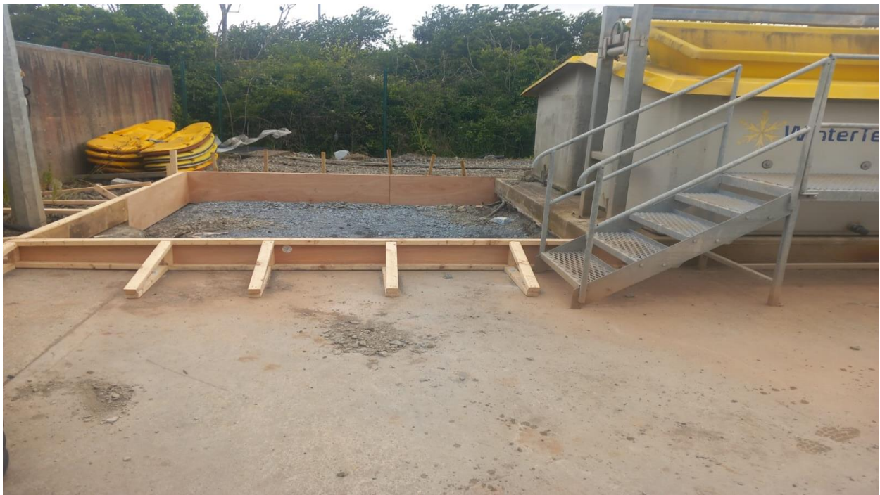
New salt silo being constructed at Faughart
