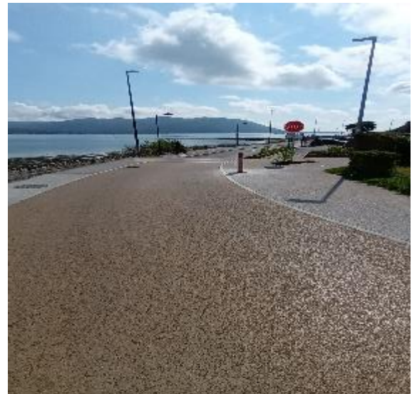
Surfacing Works Nearing Completion
