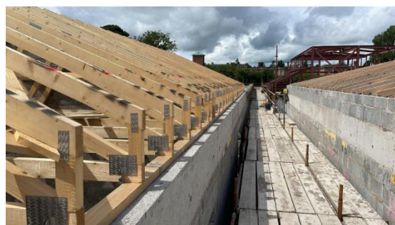
Roof Trusses installation
