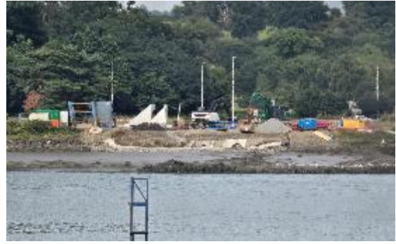
Culvert Works Northern Approach.
