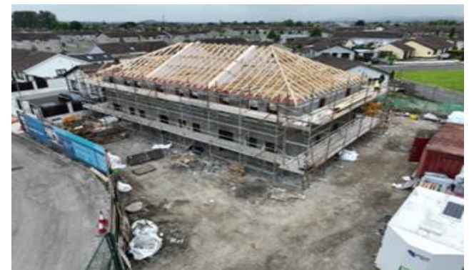
3D Concrete Printing Pilot Project at Grange Close, Dundalk
