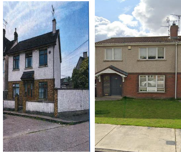
Recently acquired properties in Dundalk
