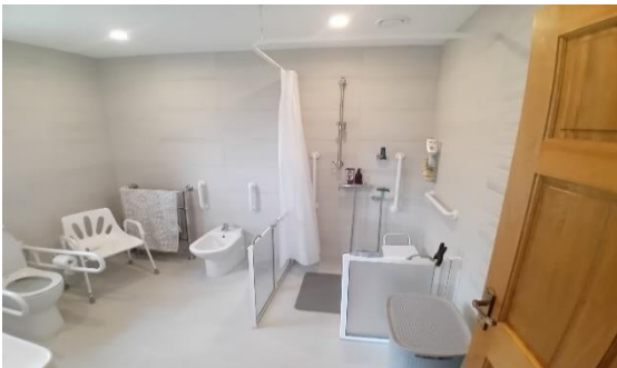
Before and after photos of a Bathroom Adaptation in South Louth part-funded by Housing Adaptation Grant
