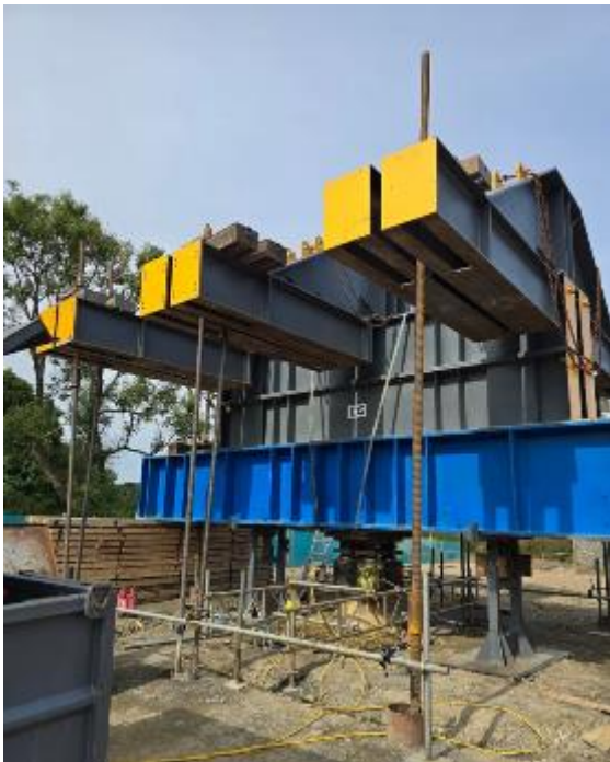
Static Load Test on Test Pile.
