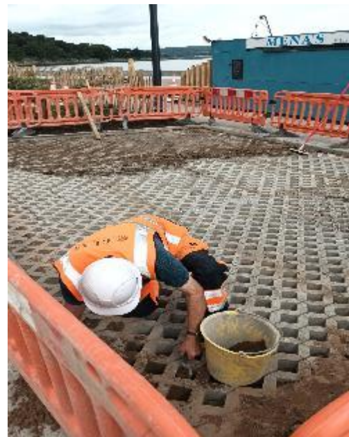
"Grasscrete" works ongoing
