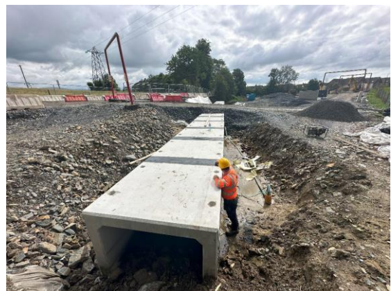
Culvert installation at Lisnawully Farm
