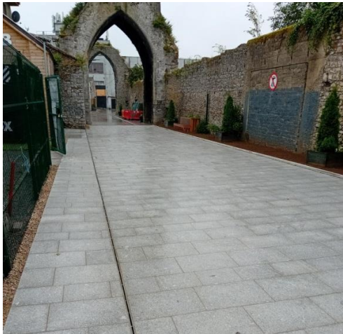
New paving works at the Old Abbey
