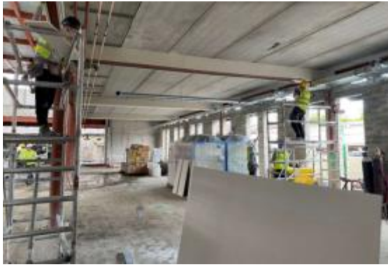
Block N: Installation of M&E and Pumping, Encasement of Steel Beams
