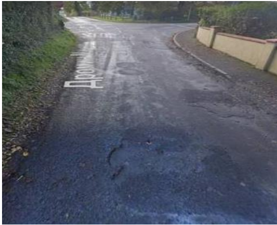
Dromin school (before)
