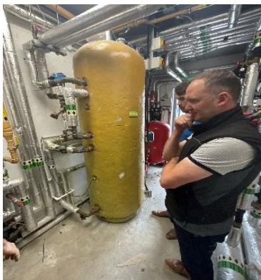
Planning new energy saving opportunities at Drogheda Fire Station
