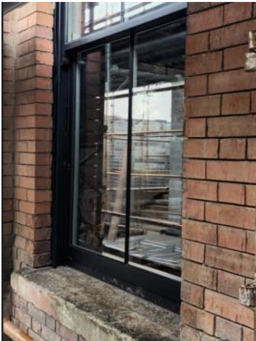
Block C: Refurbished Windows Delivered and being installation (Exterior)
