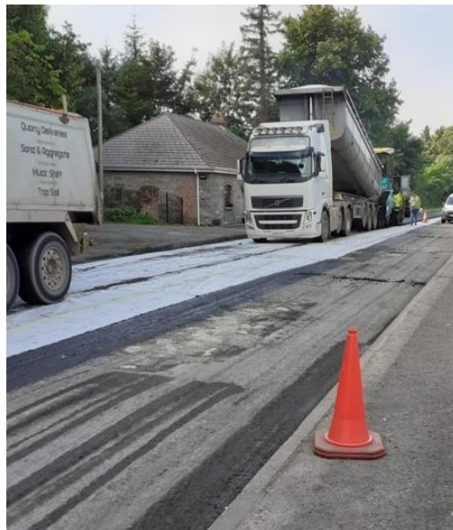
Road resurfacing works at Ardee road, Dundalk
