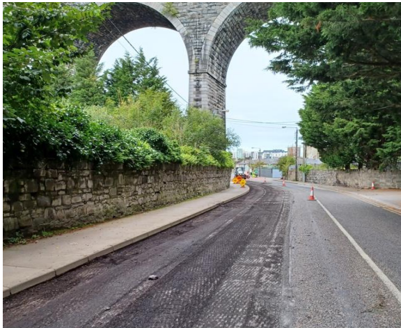
Roadworks on Marsh Road, Drogheda,
