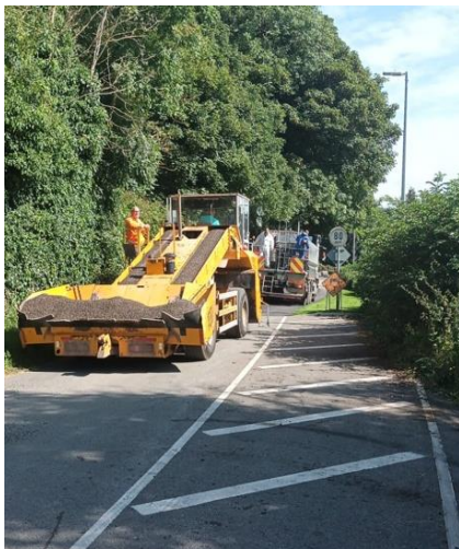
Works at Green road, Louth Village
