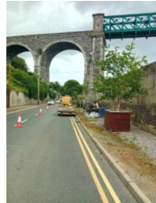
Ground Investigation works Drogheda Flood Relief Scheme
