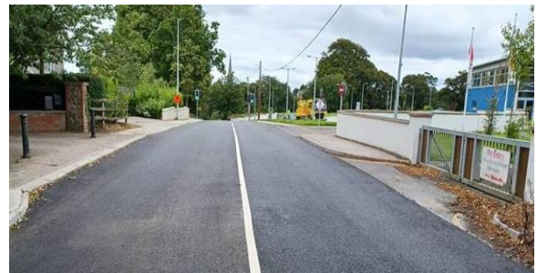
Road resurfacing at Termonfeckin, Co. Louth
