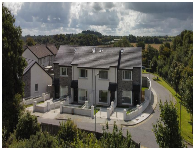
Doire Beag, Collon, Co. Louth – completed 3 bed terraced units
