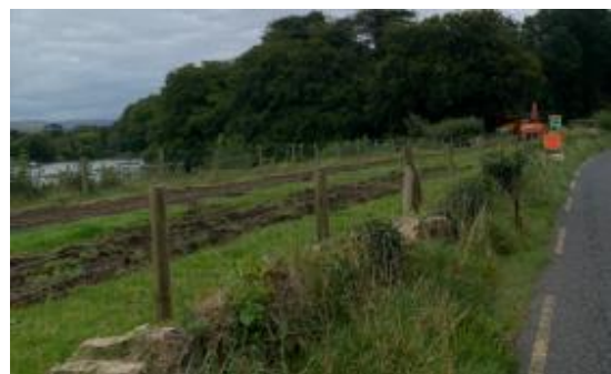
Commencement of topsoil strip
