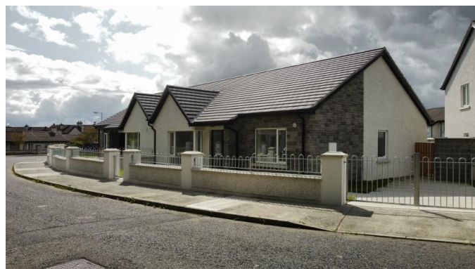
Doire Beag, Collon, Co. Louth – completed 3 bed bungalow units
