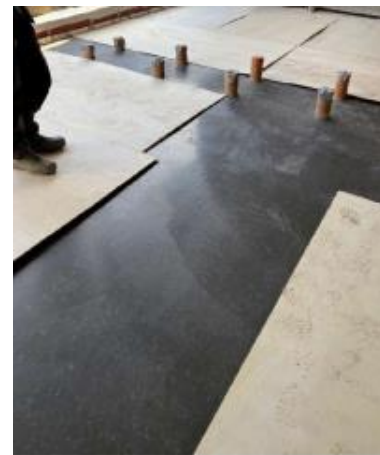
Block N Toilet Screed Sample Panel
