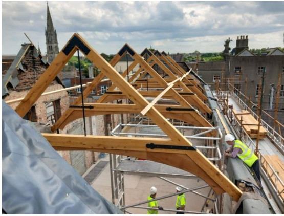
Block B – Oak Trusses and Purlins
