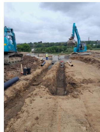
Pipework in progress Newtown
