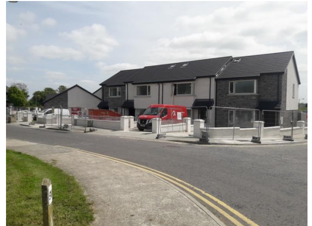
New two storey house under construction in Doire Beag, Collon
