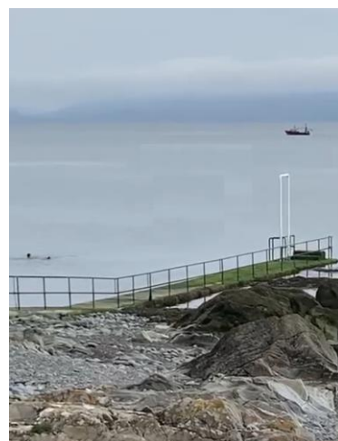
Sea weed build-up cleaned at Salterstown Pier
