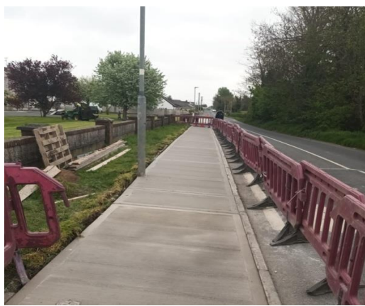
Footpath renewal at Clermont road
