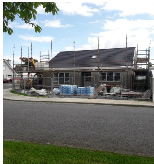
Bungalow under construction in Doire Beag, Collon.
