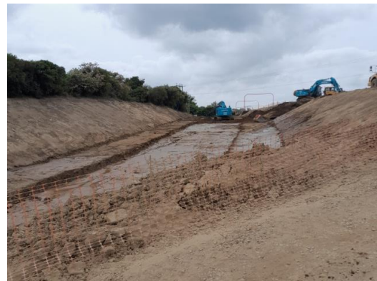
Earthworks in progress
