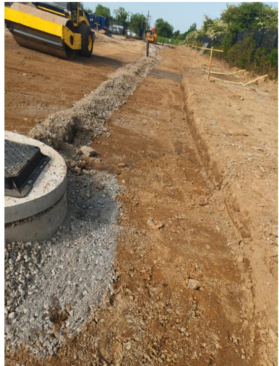
Surface Water Installation
