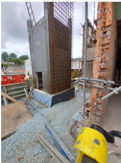
Block C Community Services Building- Lift Walls Construction
