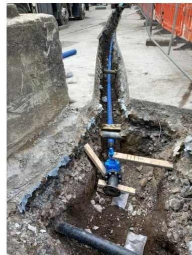
Block N New Link Building IW LCC Watermain laid.
