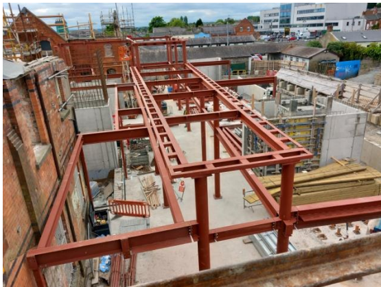
Block N New Link Building Steel Frame erection
