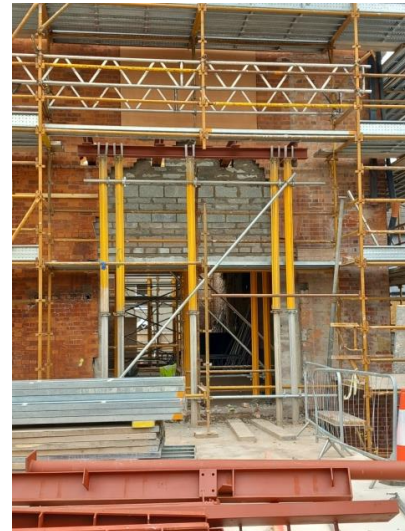
Block B Council Chamber Building- North Elevation Opening formed and Structural Steel and build up completed.
