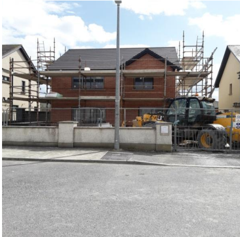
New infill housing unit under construction in Gor Uaine, Clogherhead
