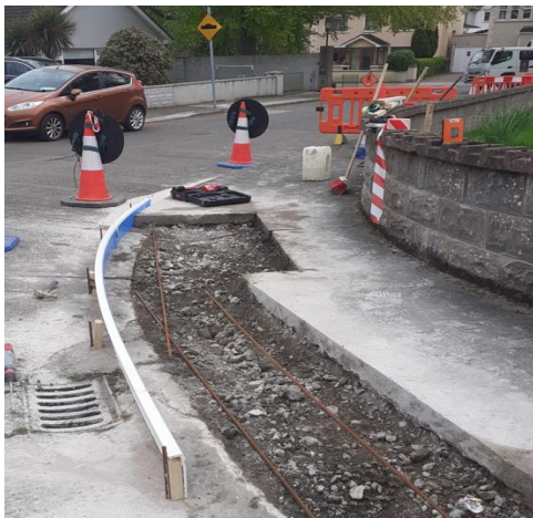
Footpath works at Ballymakenny Road
