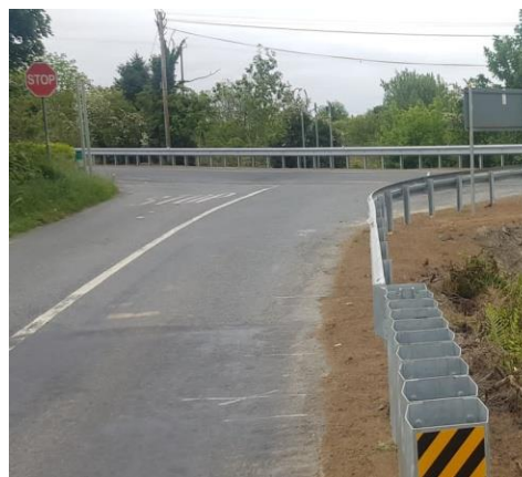
Safety barriers installed on N53
