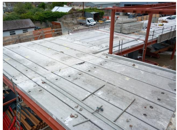
Block n New Link Building- Hollowcore Slabs
