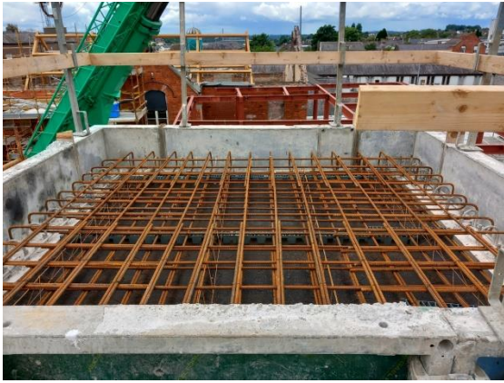
Block C Community Services Building- Lift Roof Slab Construction
