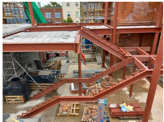
Block N New Link Building- Stairs and hollowcore slabs
