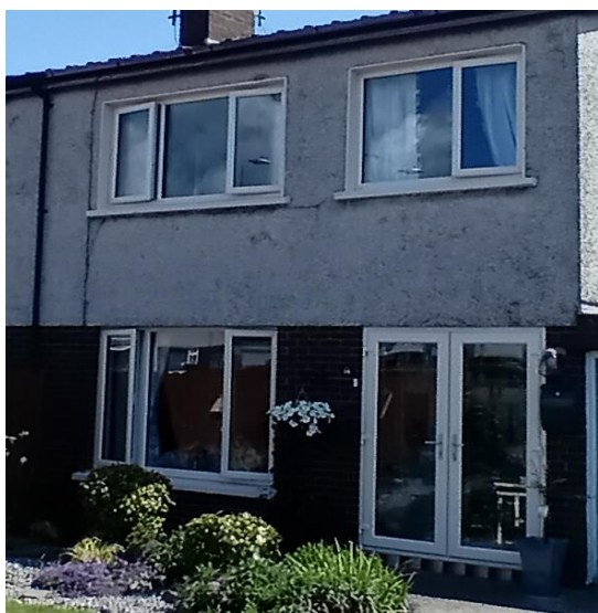
New Windows and Door completed in June with the assistance of a grant under the Housing Aid for Older People
