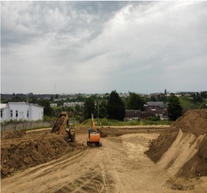
Boice Court Phase 2 – 72 unit housing Scheme commenced construction.
