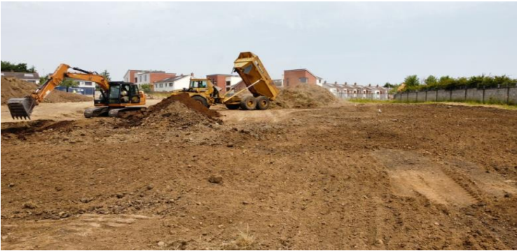
Boice Court Phase 2 – 72 unit housing Scheme commenced construction.
