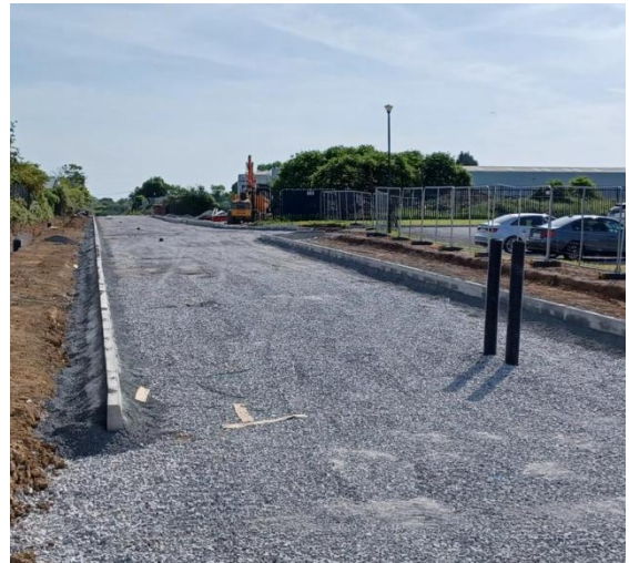
Works on the Boyne Business Park Link Road
