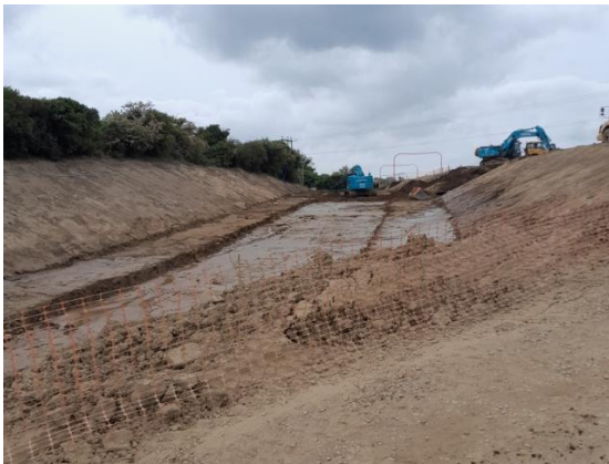
Earthworks in progress
