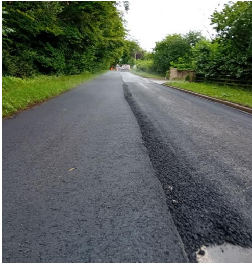
Kilsaran Works on the LP LS-6280 Bellcotton and LP-2275-24 Harestown Roads
