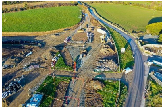
Ballymakenny roundabout construction
