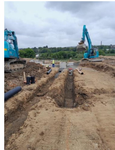
Pipework in progress Newtown
