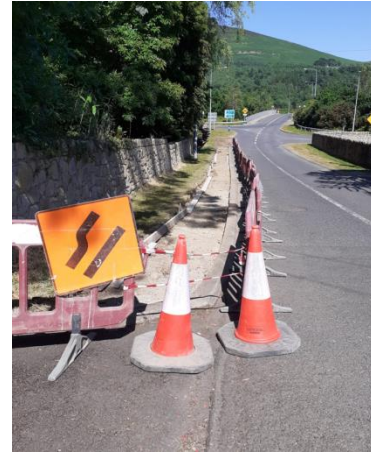
Works at Feede Loop
