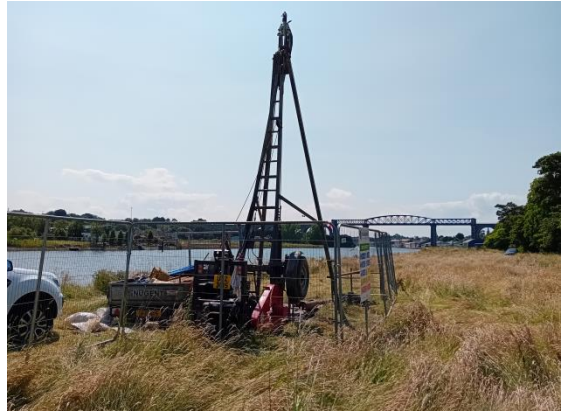
Ground Investigation works Drogheda Flood Relief Scheme
