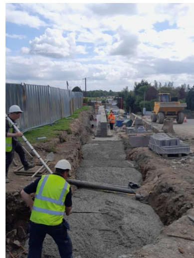
Boundary Wall construction
