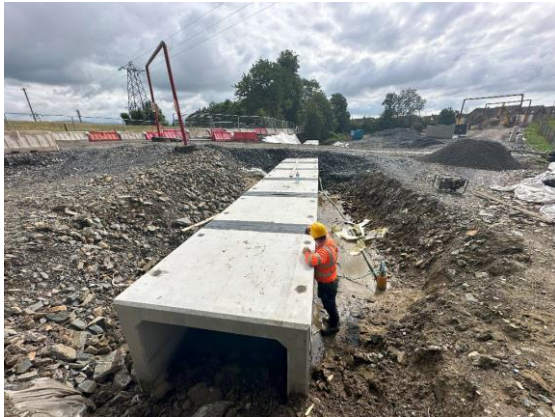
Culvert installation at Lisnawilly Farm
