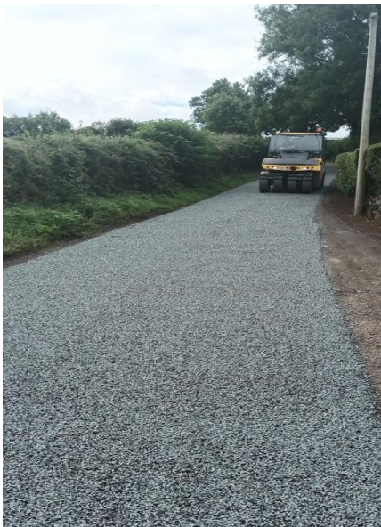
Road works in Louth Village
