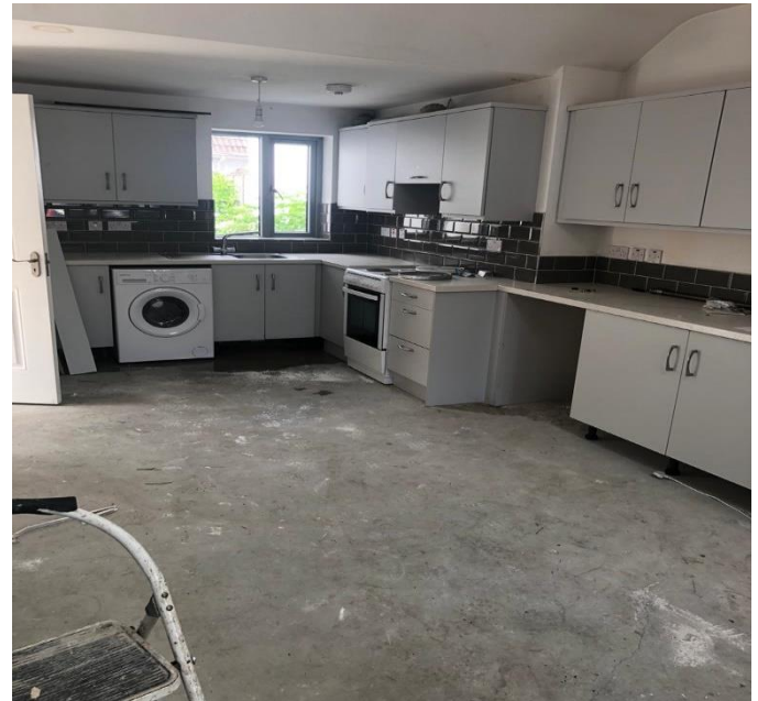
Work in Progress in a house in Ardee
