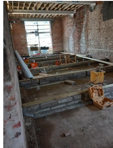
Block B Council Chamber Tassel Wall and floor joist construction
