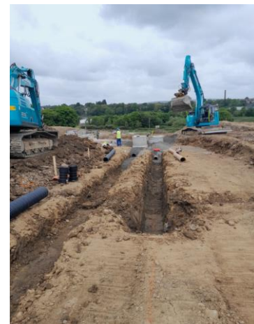
Pipework in progress Newtown
