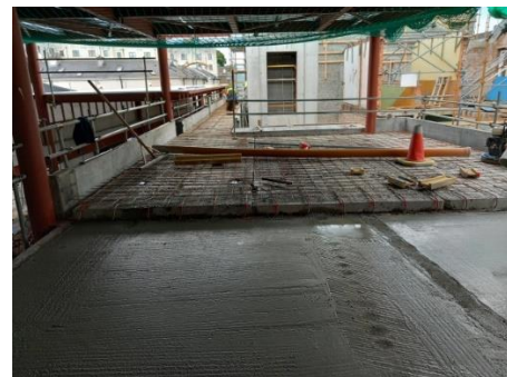
Block N New Link Building First floor hollow core screed pour
