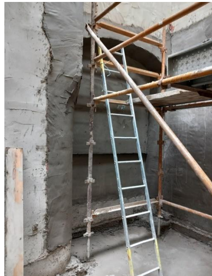
Block E Annex parge coat application
