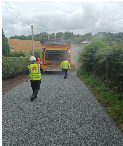
Road works at Knockabbey to Springhill
