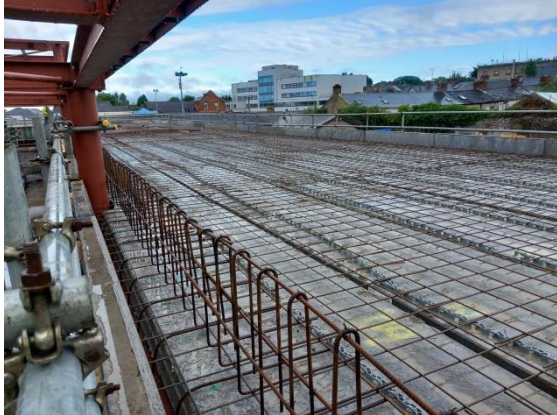
Block N New Link Building- Hollow core screed and upstand steel
