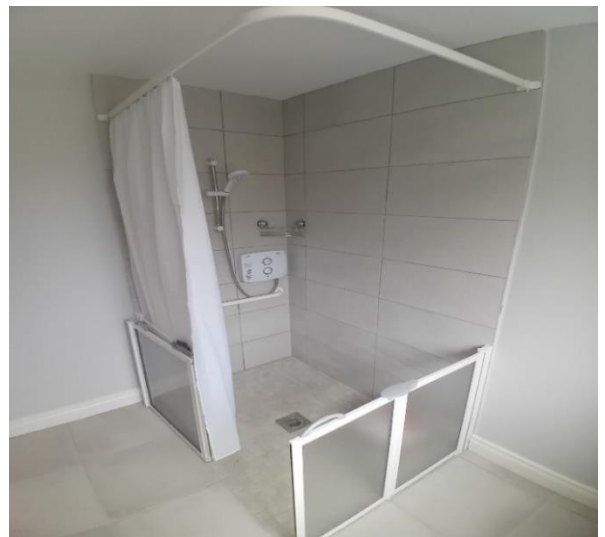
An extension for a ground floor bedroom and bathroom completed in July in Dundalk, which received funding under the Housing Adaptations Grants for Disabled.
