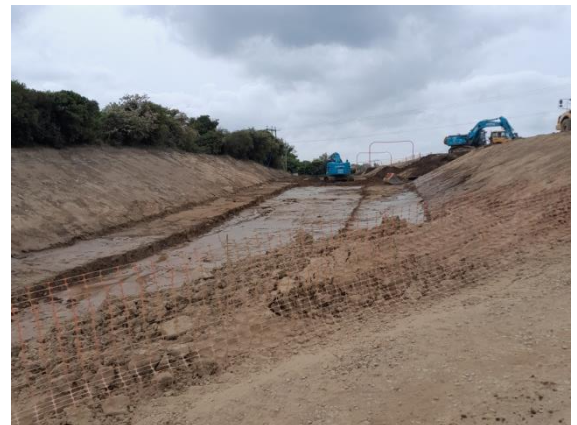
Earthworks in progress
