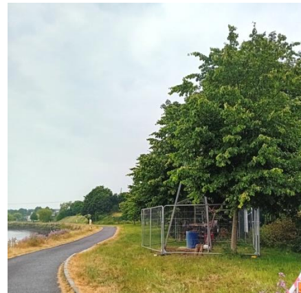
Ground Investigation works Drogheda Flood Relief Scheme
