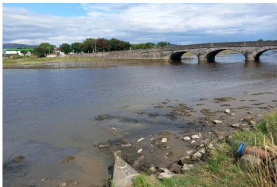
Clean-up of Castletown River, Dundalk (After)
