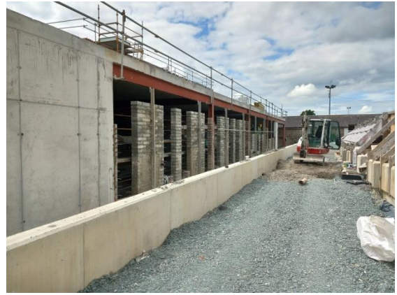
North Elevation inner leaf blockwork construction Block N New Link building
