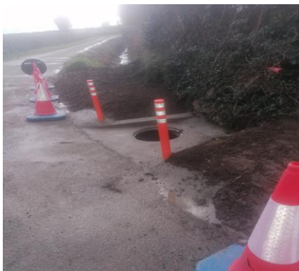
New drain constructed at Sheepgrange
