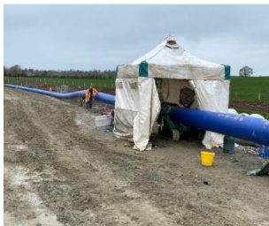
Node 2, Welding of 500mmPE SDR17 (440mmID) pipeline ongoing on site
