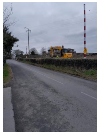
Site Clearance and Top Soil removal
