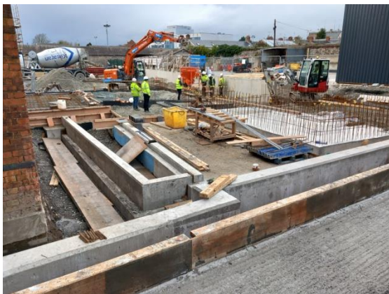
Block N Eastside Ground Beams & Slabs
