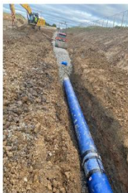
Node 2, Welding of 500mmPE SDR17 (440mmID) pipeline ongoing on site
