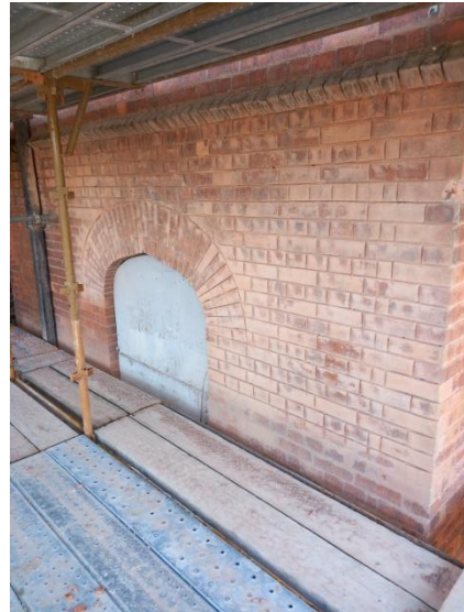
Block B – Raking out brickwork for repointing.
