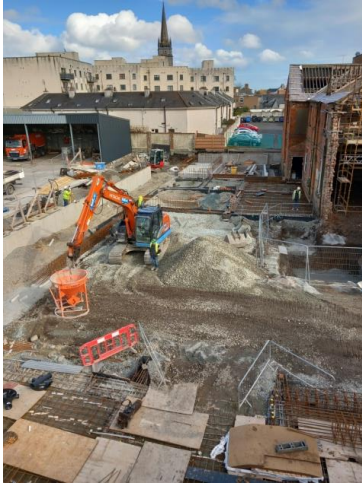
Block N New Link Building Construction Works
