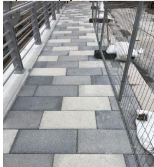
Upstream South elevation footway paved
