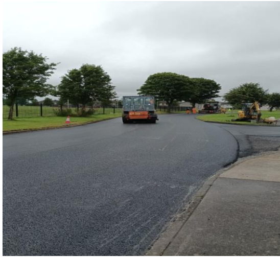
Resurfacing at Slieve Foy Park
