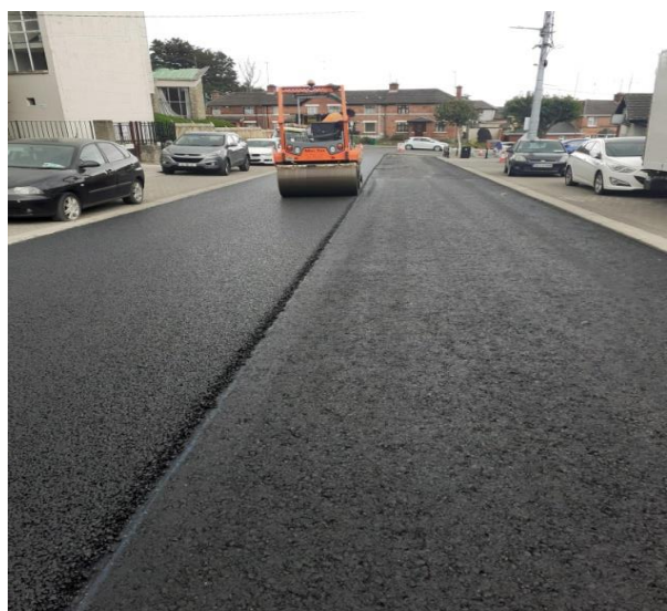
Resurfacing at Bothar Brugha
