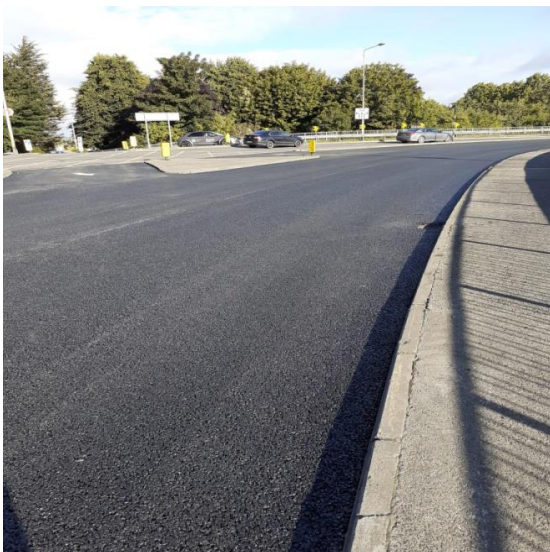
Resurfacing at Dual Carriageway
