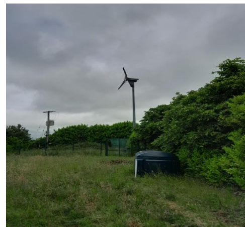
Turbine at Louth County Council Dog Pound, promoting renewable energy.
