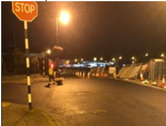
Night time works to resurface the junction
