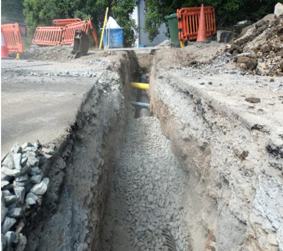
Waterunder Culvert Repair
