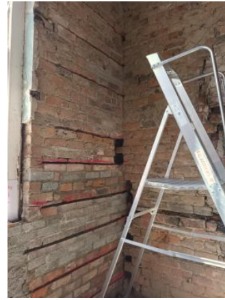
Stitching works to stabilise brickwork in Block C
