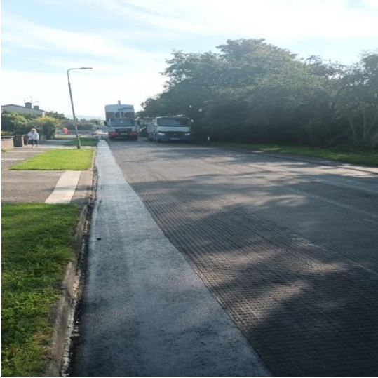
Installing of Geo Grid at Greenacres
