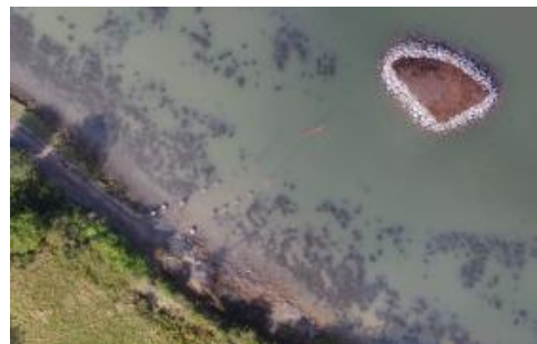
Completed Roost Site Works
