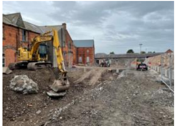
Removal of Spoil from Piling mat
