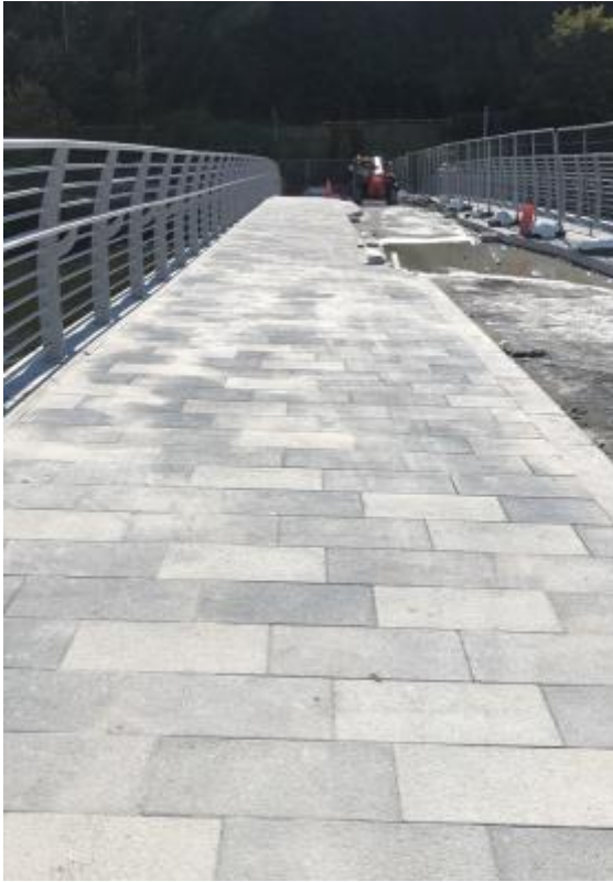
Re-laid Paving on Port Side of the Bridge
