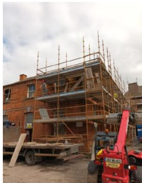
Scaffolding Erection at Block C to enable Demolition
