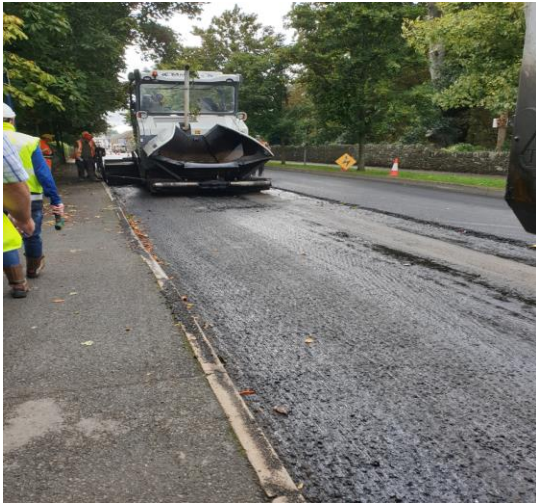
Road Resurfacing on the LP-1233-7 Townspark Ardee with the N2
