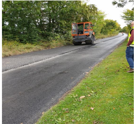
Road Resurfacing on the LS-6274-0 Gallstown
