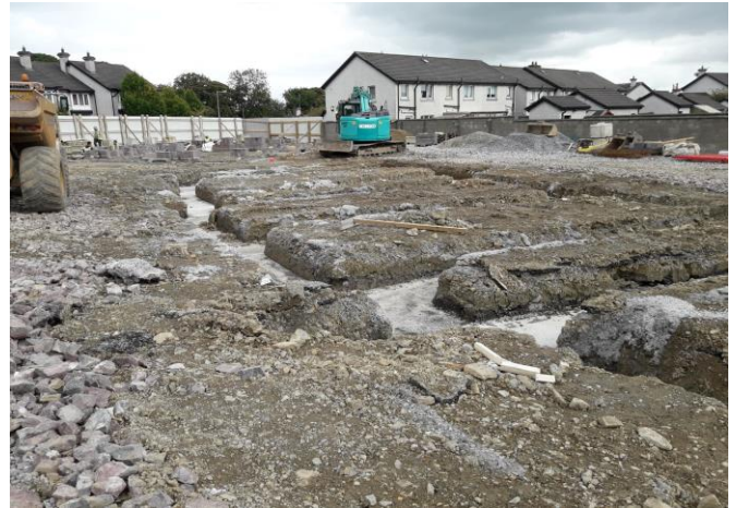
Foundations for new housing units – Doire Beag Phase 2C
