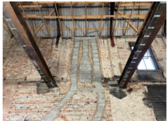
Infill of Chimney Flues in Block E
