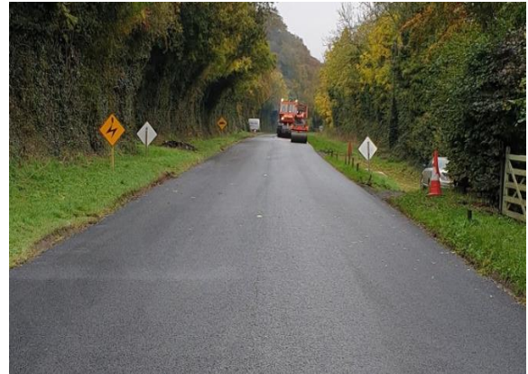
N51 Resurfacing Works
