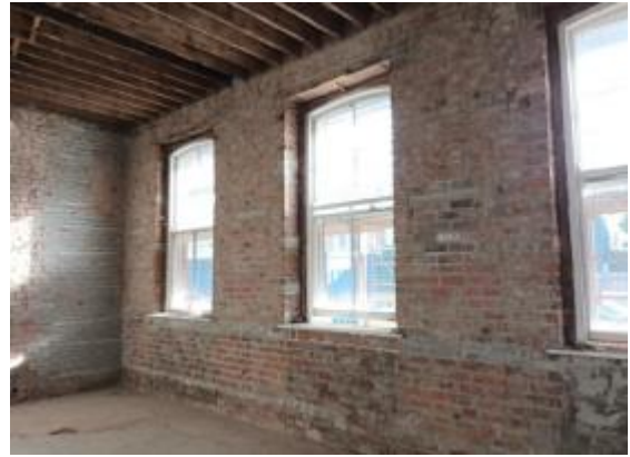
Complete repaired panels Block C
