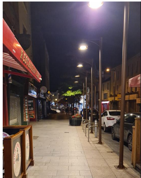
New Street Lighting at West Street, Drogheda
