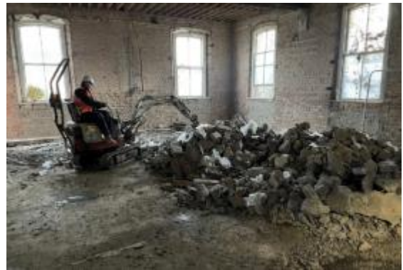
Demolition of the Floor Slab Block C
