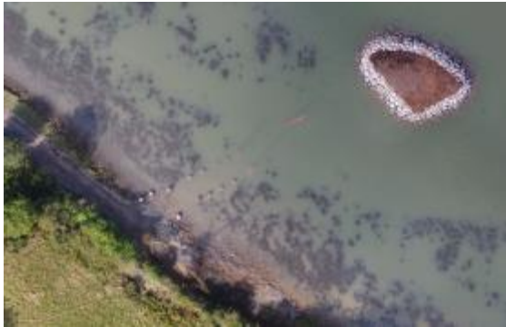
Completed Roost Site Works
