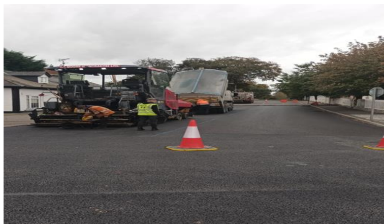
Road repairs at Tallanstown
