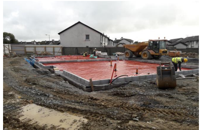
Sub-Floor works for new housing units - Doire Beag Phase 2
