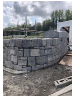
St. Dominick's Bridge- Wing-wall rebuilt
