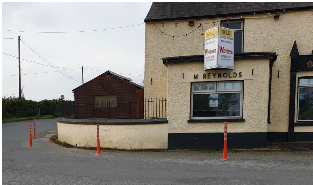
Bollards installed at Stabannon junction
