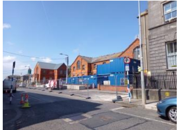
Contractor setting up compound
