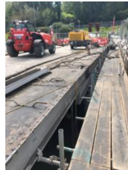
Steel Deck Exposed
