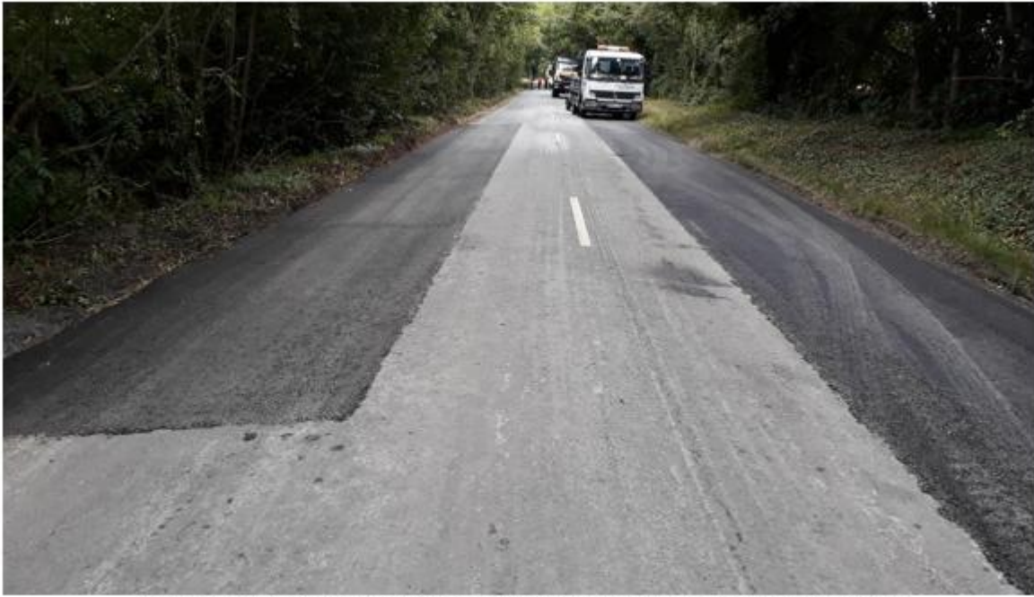
Edge Strengthening on Carstown Road prior to Surface Dressing
