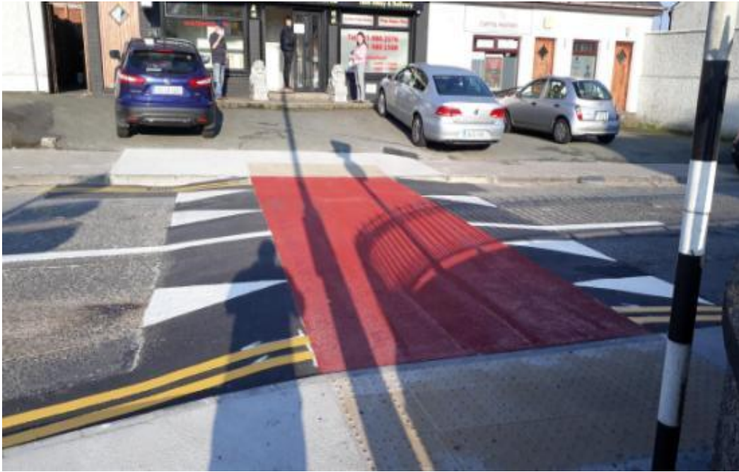
New Raised crossing at top of King Street, Drogheda. One of five new raised crossings to enable Schoolchildren to cross safely in the vicinity of St. Joseph's National School and promote "Active Travel"
