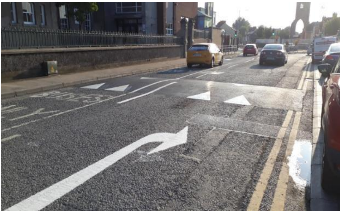
New Speed ramp on approach to St. Joseph's Primary School, Sunday's Gate
