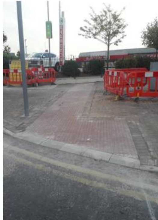
Construction of new Pedestrian Crossing at Kierans Corner
