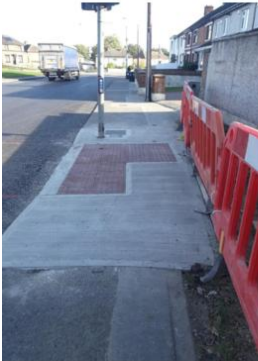
Up-grade of Pedestrian Crossing at Platin Road
