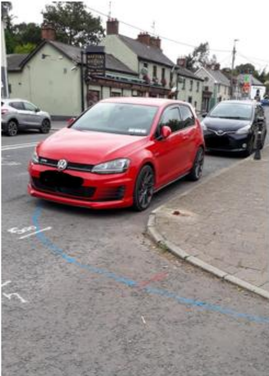
New kerbline position in Collon village to prevent cars parking at junctions and blocking sightlines
