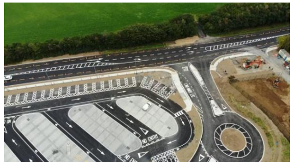
Aerial View of Park & Share Construction progress
