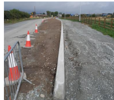
Footpath & Cycle Lane Construction Progress
