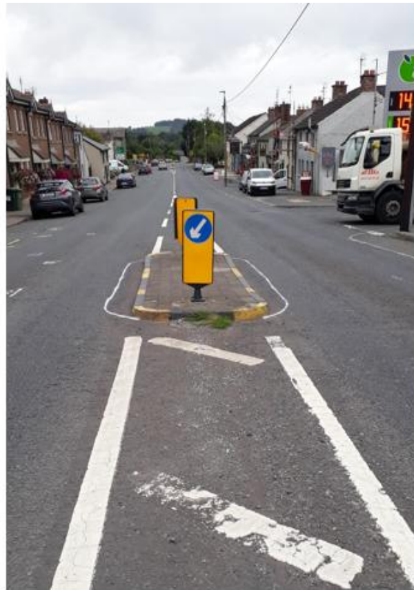
Collon - Line markings showing kerbline builds outs at central islands to narrow carriageway and slow traffic
