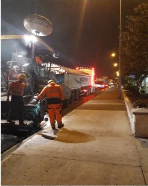
Night Work on Newry Road - RWP 2021
