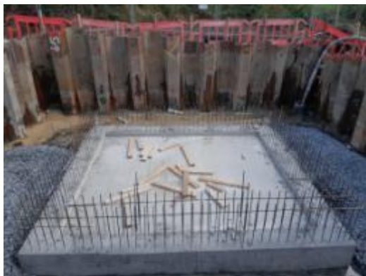
Base Slab of Inlet Chamber
