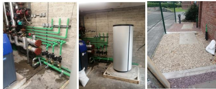
Works for the New Air Source Heat Pump at County Hall
