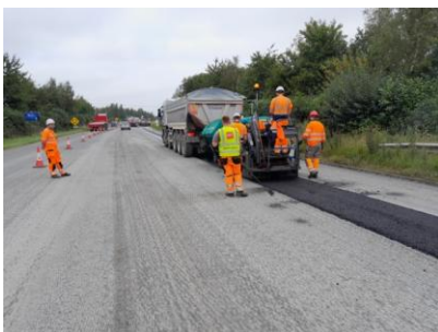
Laying of new road surface
