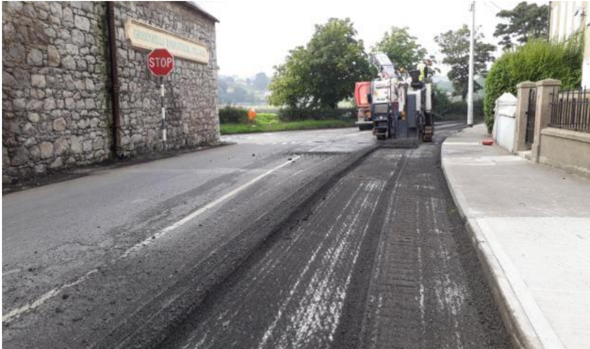
Planning out for new road surface at Ushers Corner
