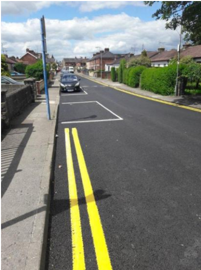
Resurfacing at Thomas Street
