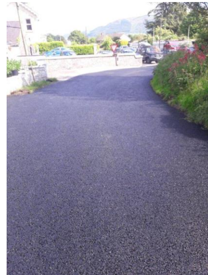
Resurfacing South Commons, Carlingford.
