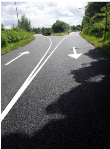
Resurfacing at Haynestown
