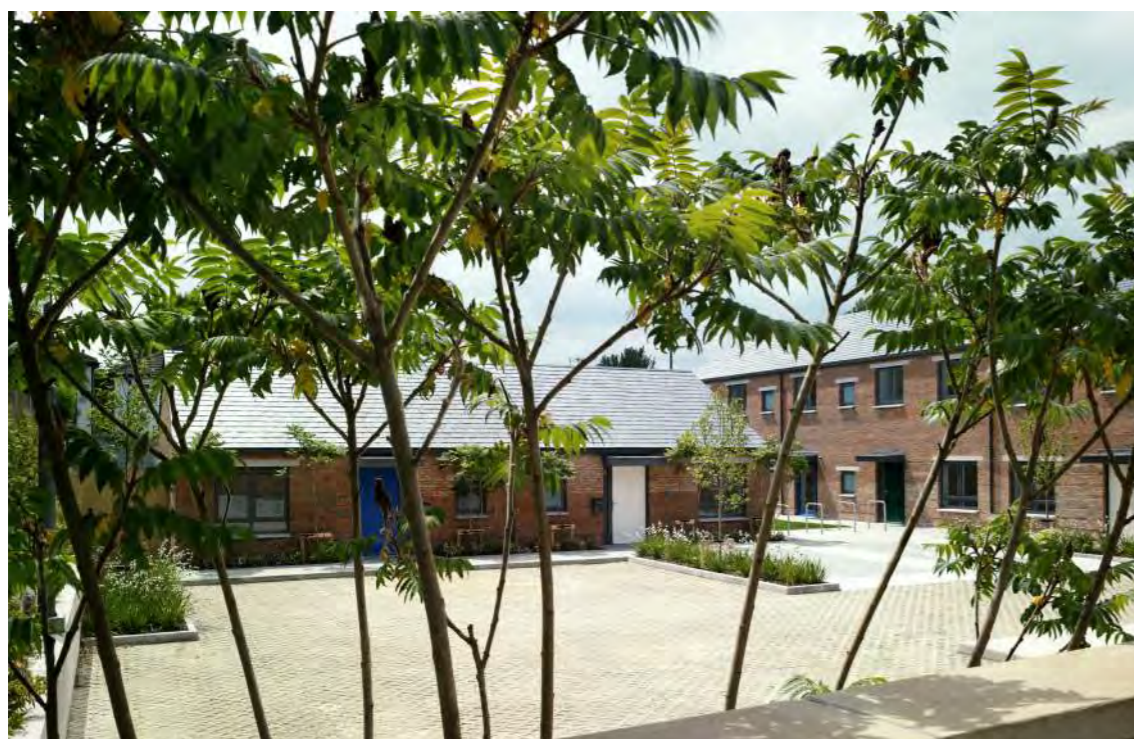
The Brambles Retirement Housing, Sallynoggin, A2 Architects
