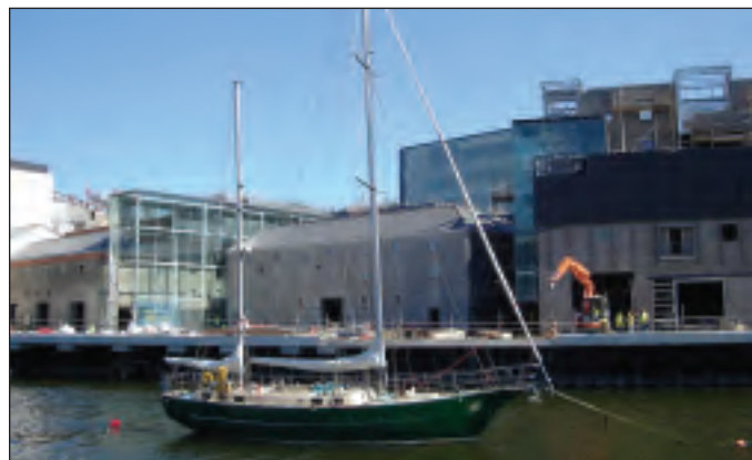
Scotch Hall will raise the standard of urban design in Drogheda and stimulate future development of the South Bank area.
