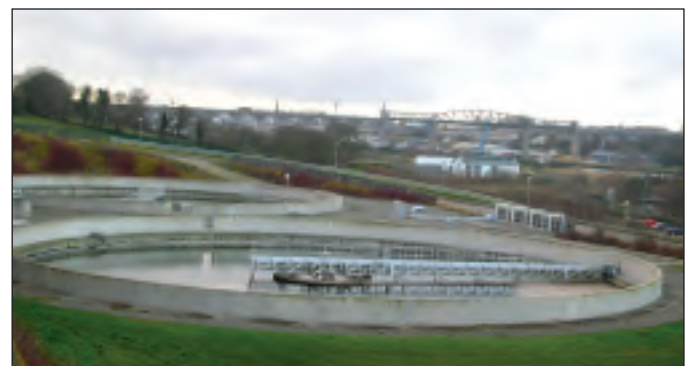
Marsh Road Wastewater Plant
