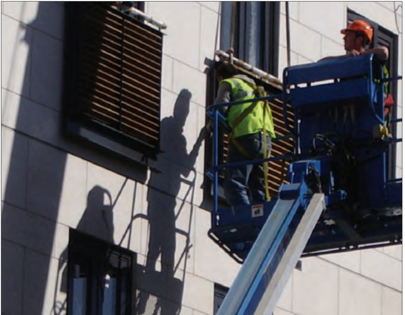
Construction of Scotch Hall
