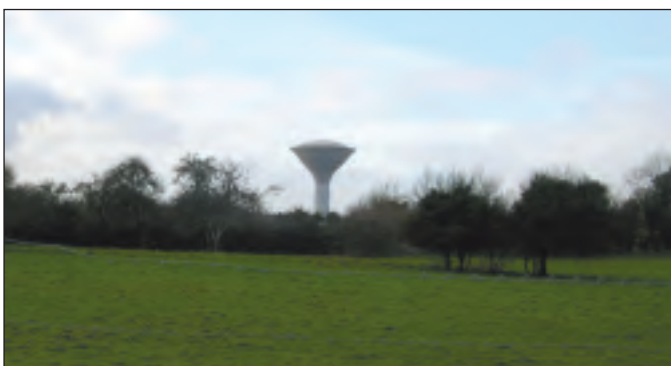
Water Storage Tower
