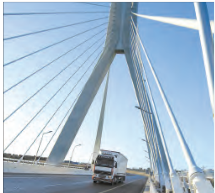
Boyne Cable Bridge
