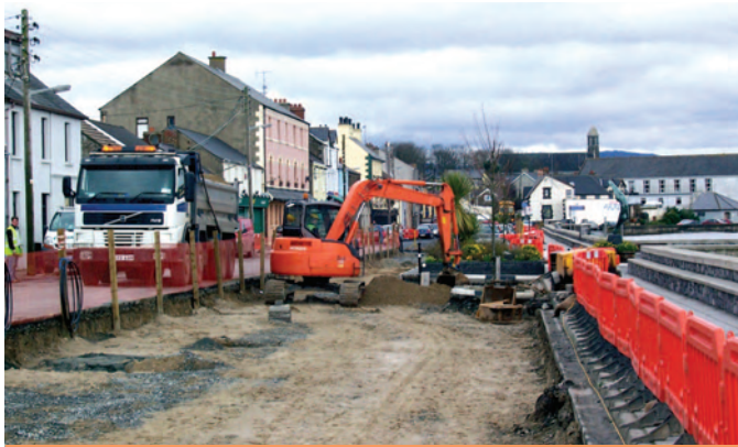
Blackrock Main Street improvements.
