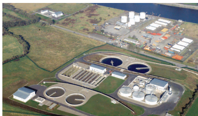
Drogheda Sewage Treatment plant.
