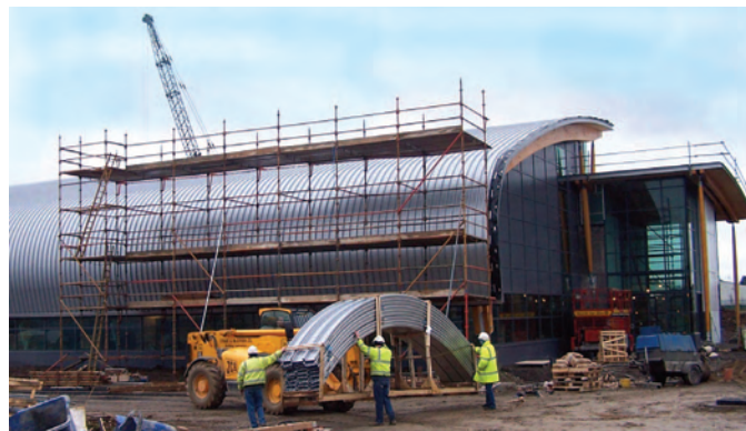
Work in progress – Drogheda Swimming Pool.
