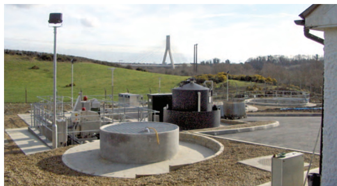
Tullyallen Sewerage Works.
