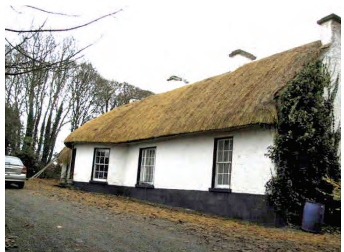
Rethatching a cottage at Whiterath.
