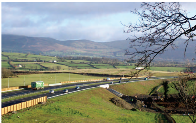
Dundalk Western By-pass open to traffic.
