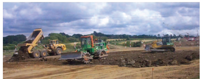
Dundalk Western Bypass under construction
