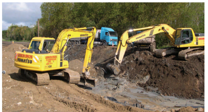
Rockmarshall Improvement Scheme – installation of box culvert
