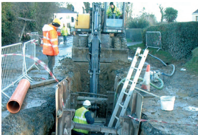
Pipe laying – Baltray Termonfeckin Sewerage Scheme
