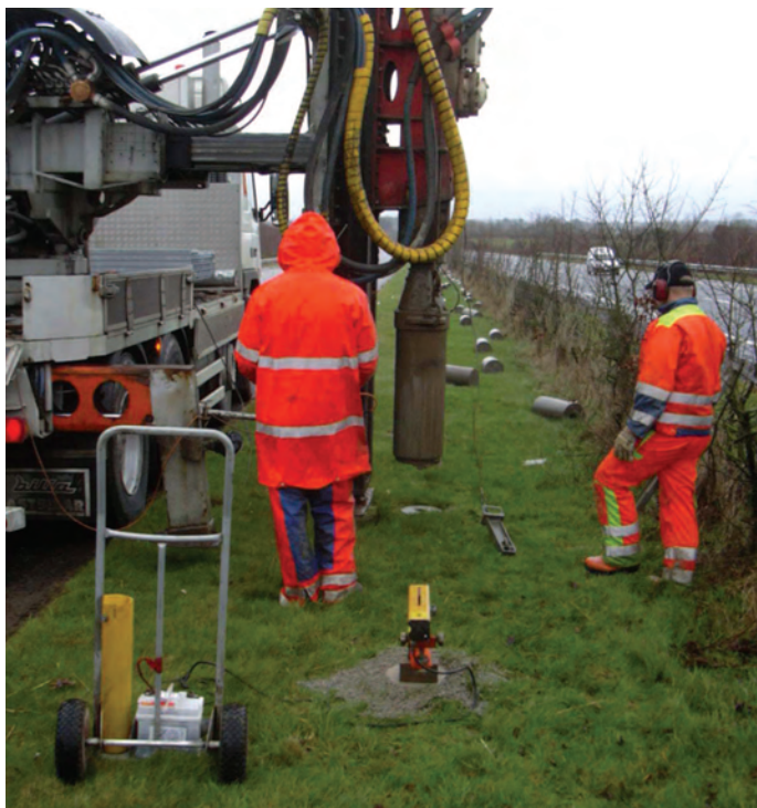
Retro-fitting Median Safety Barrier on M1
