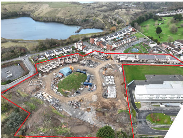
Boice Court, Mell, Drogheda. Construction commenced in 2023. 72 Units
