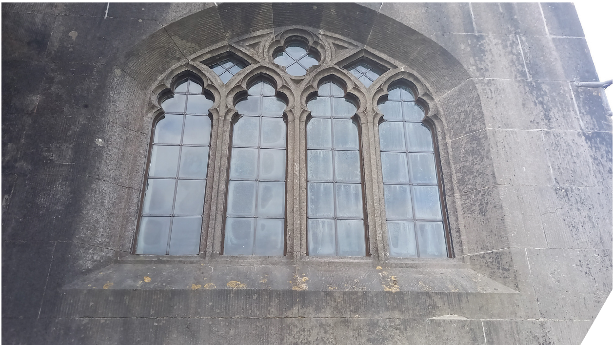
Collon Church North Window re-glazed and re-leaded
