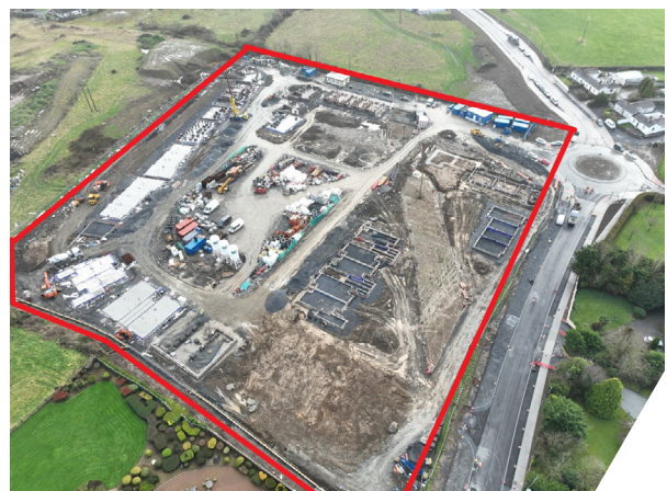
Mount Avenue, Dundalk. Construction commenced in 2023. 93 Units
