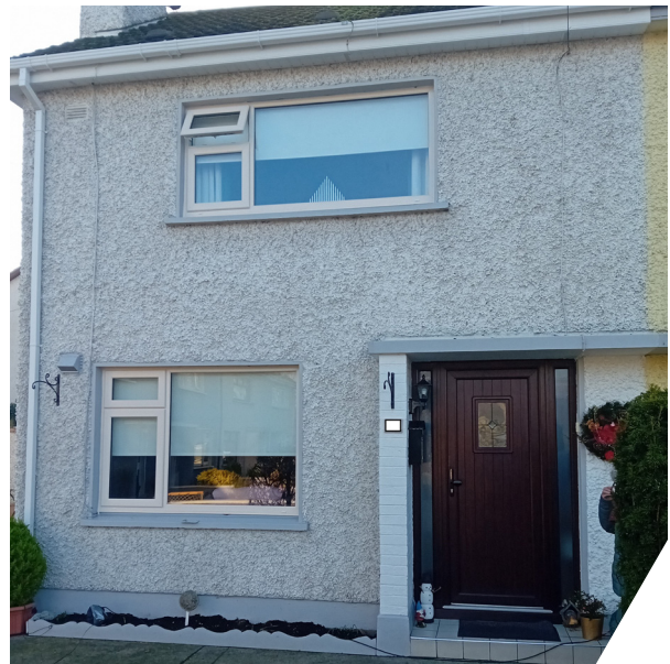
New Windows installed in a house in Tallanstown 2023 with assistance from a Housing for Older Persons Grant
