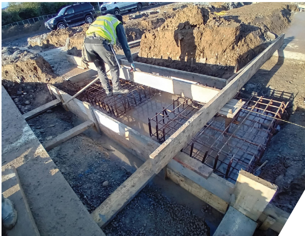
Ardee Educate together School, commencement of foundation works
