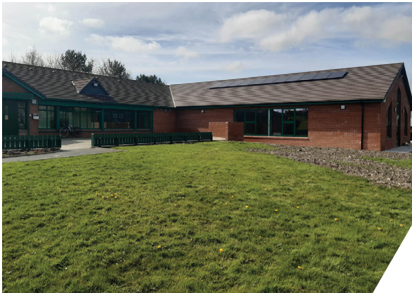
Muirhevnamór Community Centre Extension, Dundalk
