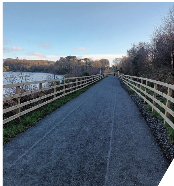
Carlingford Lough Greenway Completion of final Surface at the Border
