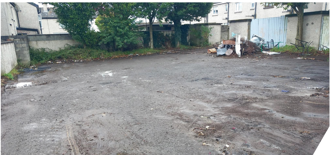
Muirhevnamore Alley Clean up – After completion of works
