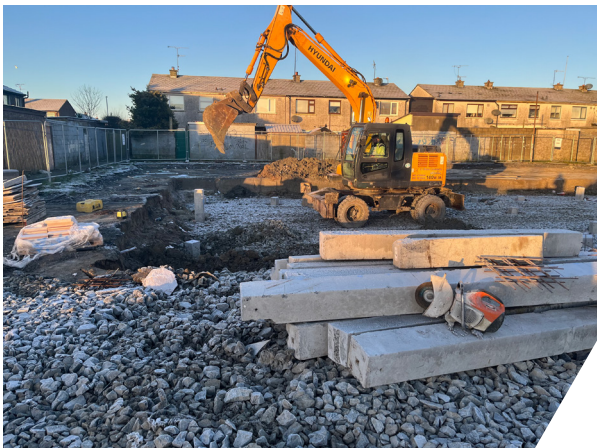
Muirhevnamór, Dundalk. Construction commenced in 2023. 11 Units
