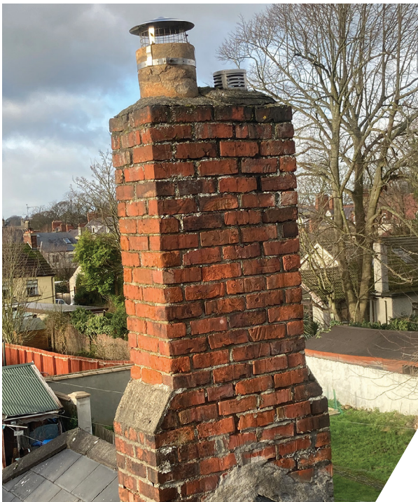
Castle Road Chimney (before)
