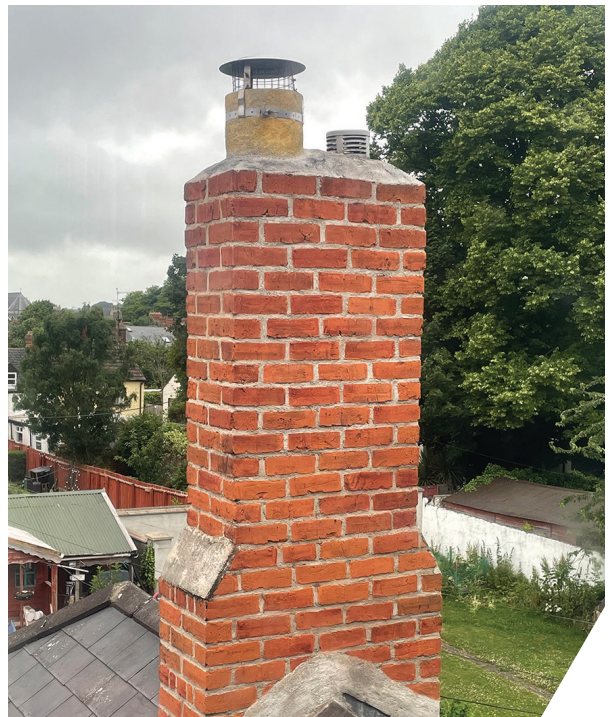
Castle Road Chimney repairs (complete)
