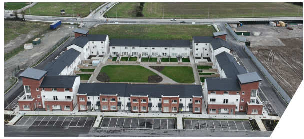
Ellwood, Ballymakenny, Drogheda. 46 Units
