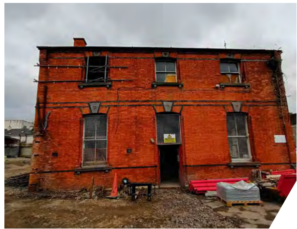
Block C Community Services Building West Elevation pre dismantling
