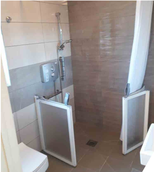
Level access shower installation using private house grant
