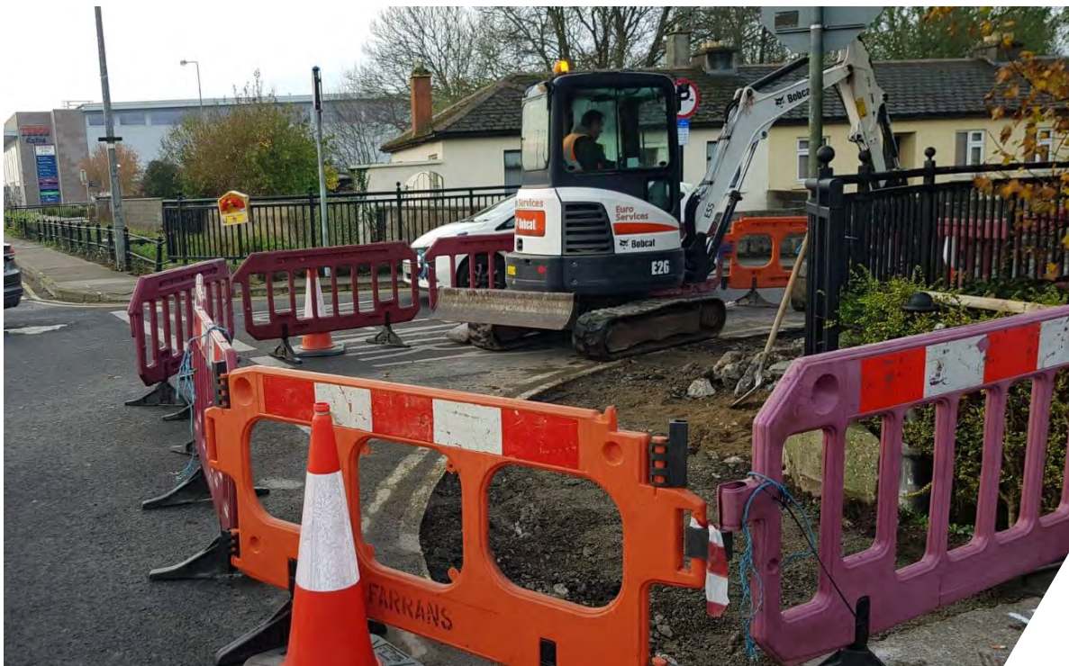
Footpath reinstatement works in Dundalk
