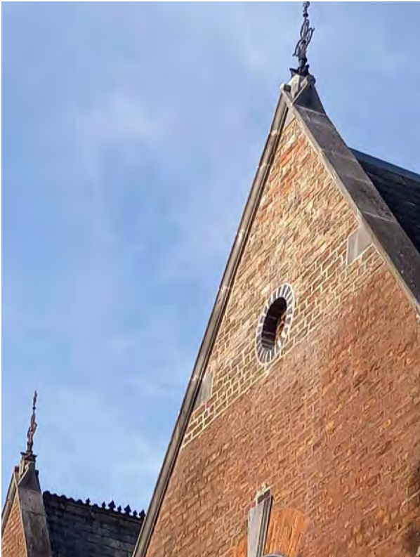
The Sycamores Capping Stone & Front Gable Rebuild
