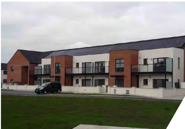
New apartment building at Patrick Tierney Crescent, Dundalk
