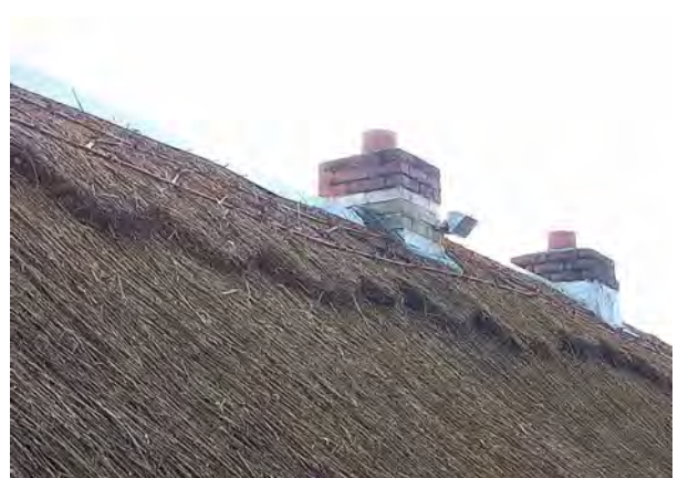
Townley Hall After
