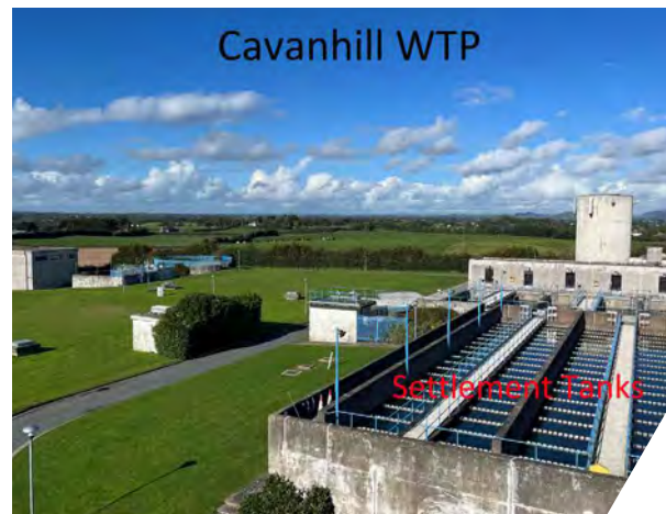
Cavan Hill Water Treatment Plant
