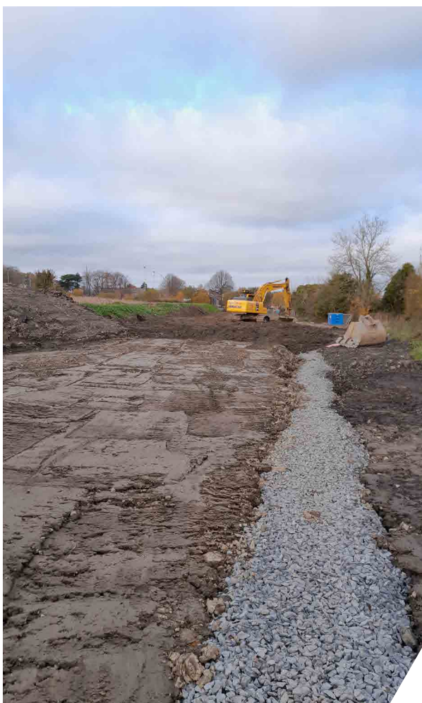
Recently completed flood alleviation works
