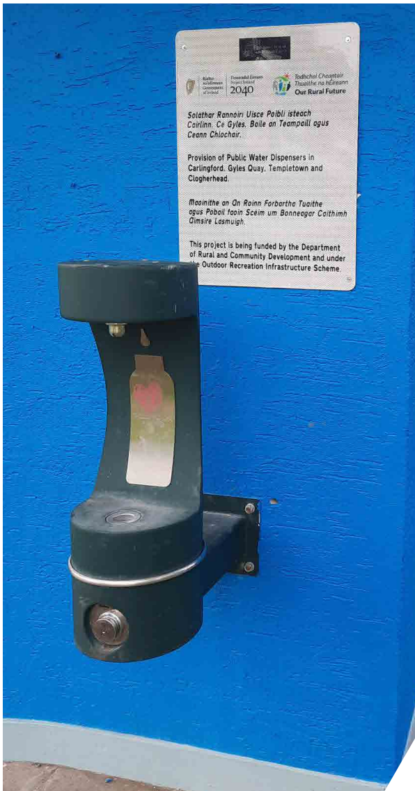
Drinking Water Station Carlingford
