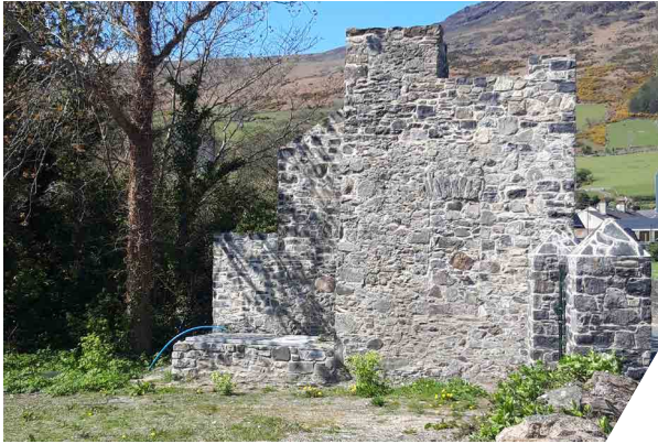
Ghan Folly Walls and Tower works
