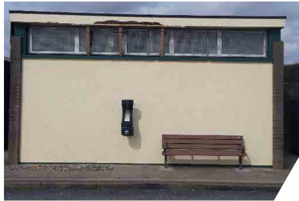
Drinking Water Station Gyles Quay
