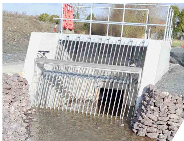
Recently completed flood alleviation works
