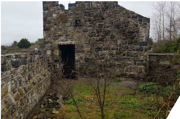
Ghan Folly Walls and Tower works
