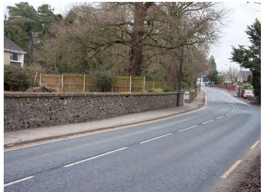
Plate 28: General view of boundary wall looking northeast.
