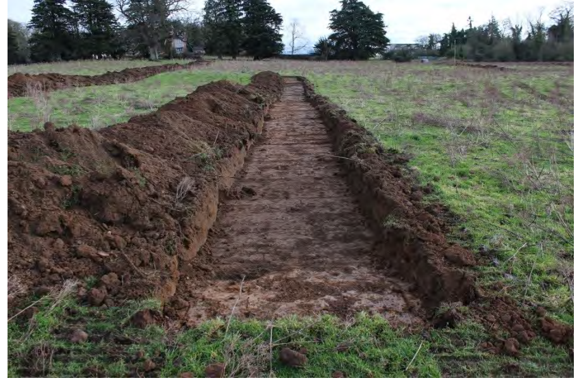
Plate 6: Trench 2. Looking east.
