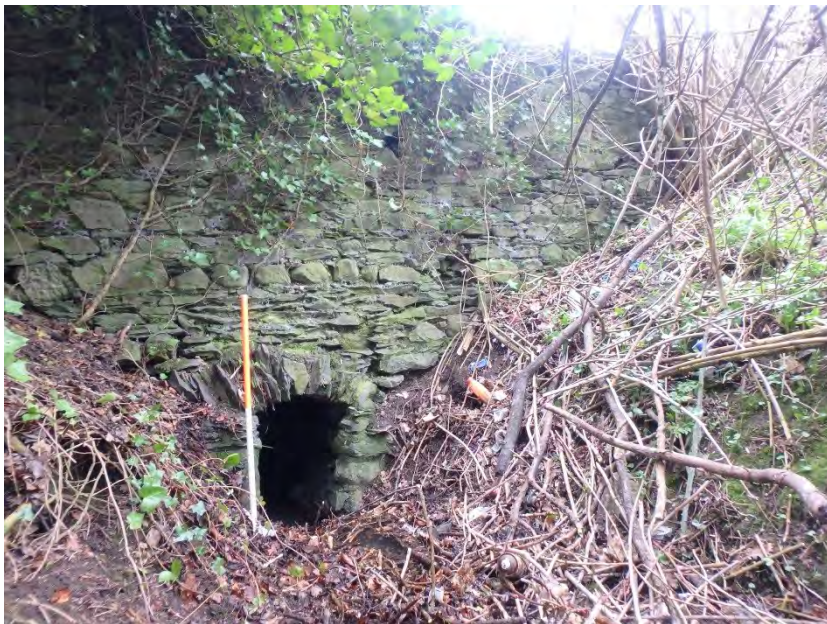
Plate 31: View of stone culvert looking southwest.
