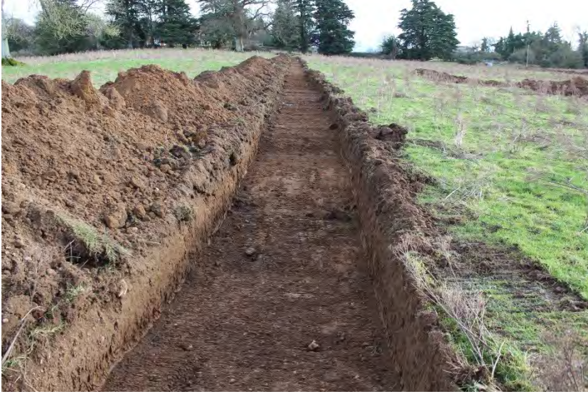
Plate 5: Trench 1. Looking east.
