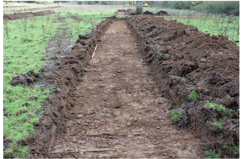
Plate 12: Trench 8. Looking east
