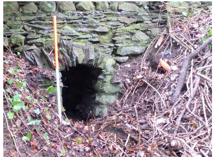
Plate 32: View of stone culvert looking southwest.
