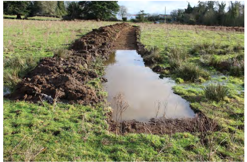
Plate 8: Trench 4 Looking east.
