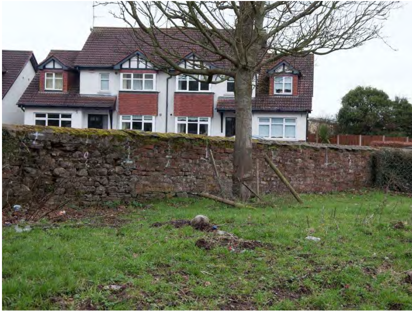
Plate 29: View of interior of wall showing brick looking southwest
