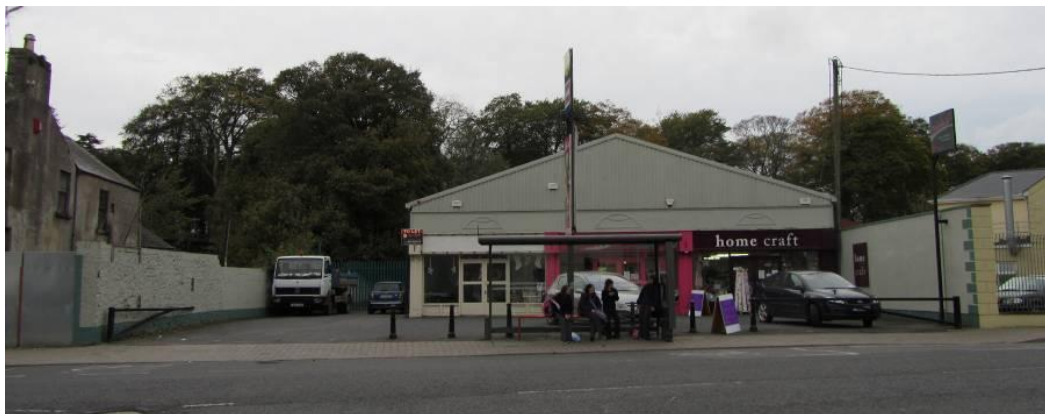
Fig. 130: New buildings which ignore the established building line and plot sizes damage the character of the street space
