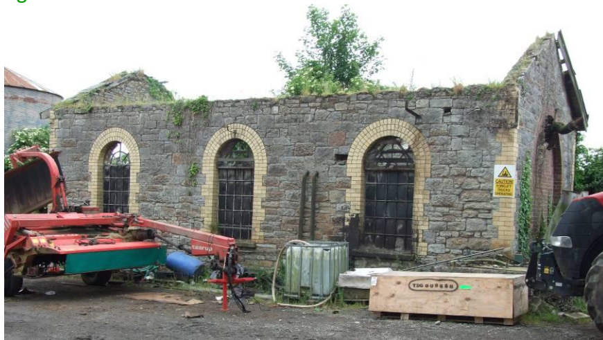
Fig. 67: Former Station Good Shed
