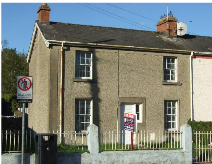
Fig. 65: End house of Railway Terrace with sash windows and railings
