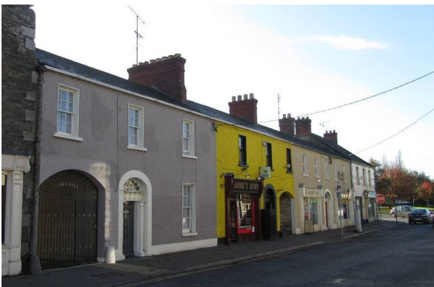
Fig. 86: Terrace of houses to the south of William Street
