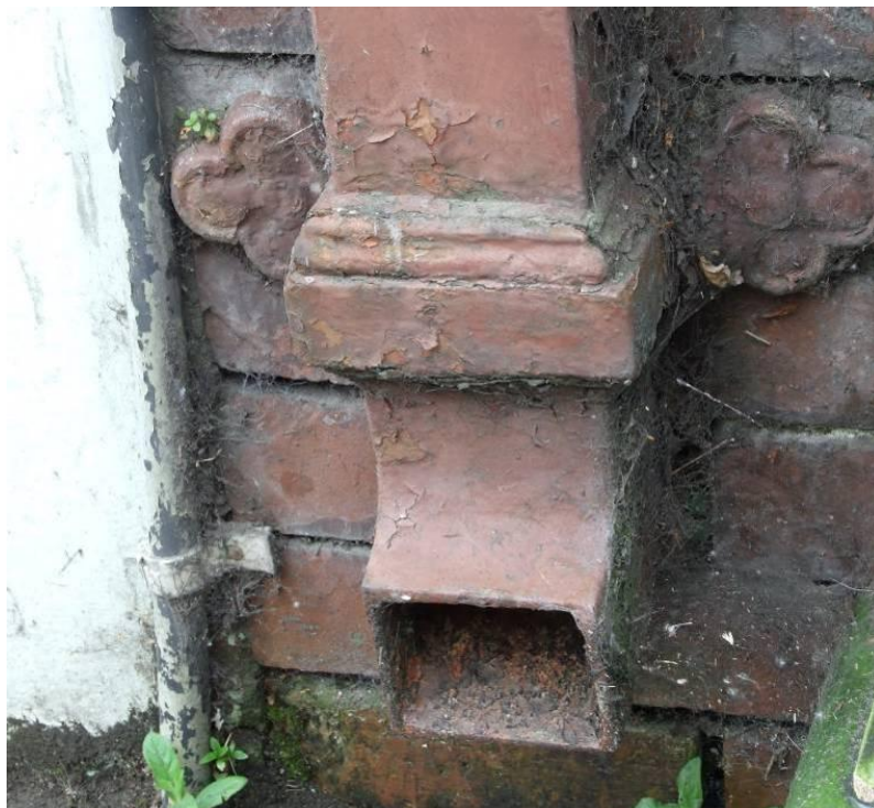
Fig. 108: Down pipe with decorative fixings, Bridge Street
