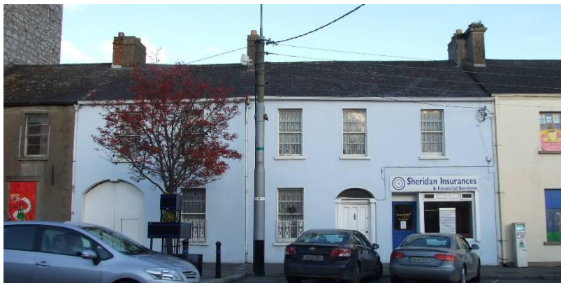
Fig. 24: Houses on east side of Castle Street
