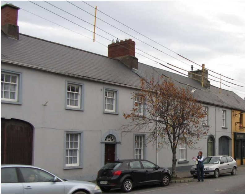
Fig. 23: Houses to east side of Irish Street
