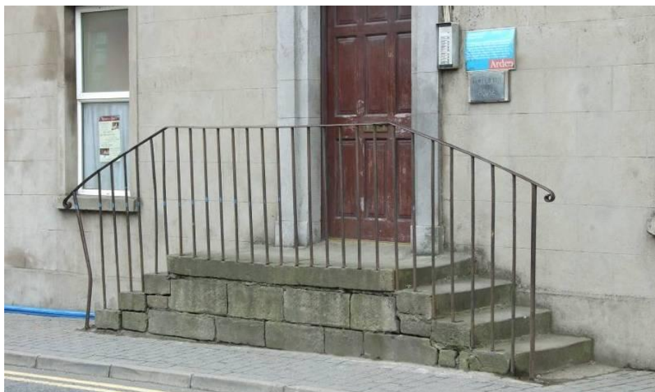
Fig. 128: Railings and steps on Bridge Street
