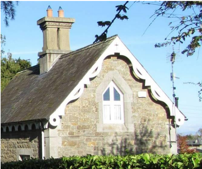
Fig. 107: Decorative bargeboards to convent gate lodge
