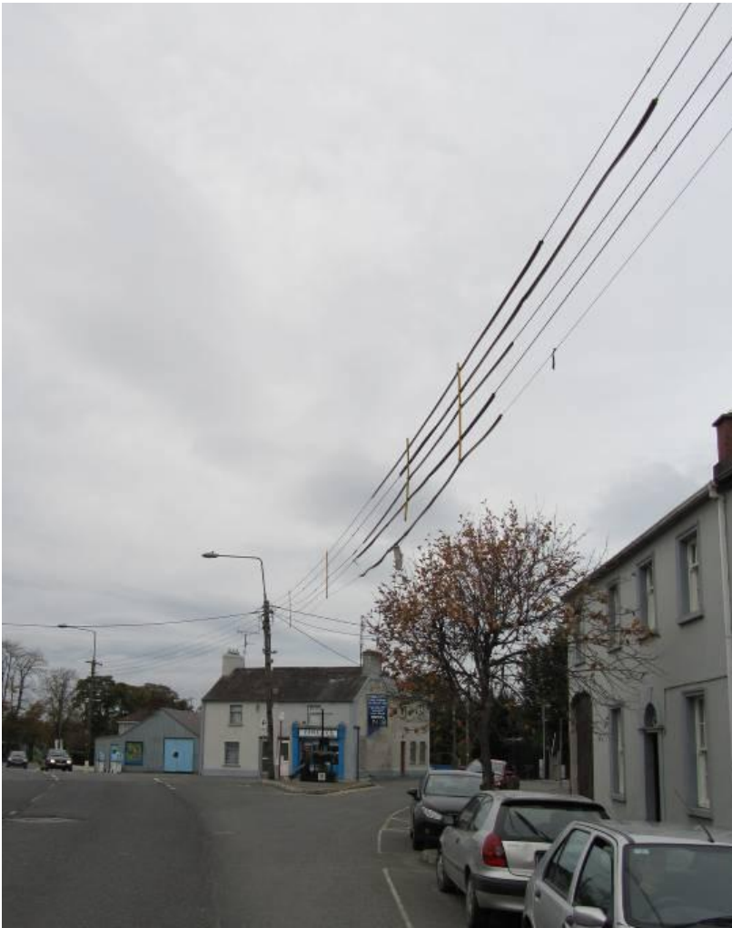
Fig. 137: Obtrusive overhead cables on Irish Street
