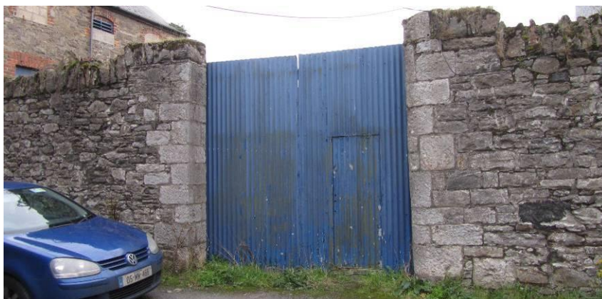
Fig. 61: Warehouses to rear of Ulster Bank, Market Street
