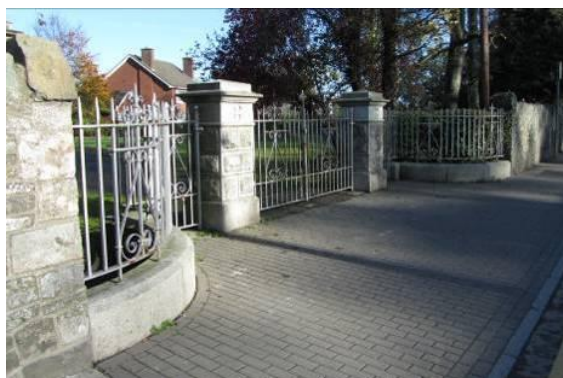
Fig. 97: right: cast iron gates and stone piers
