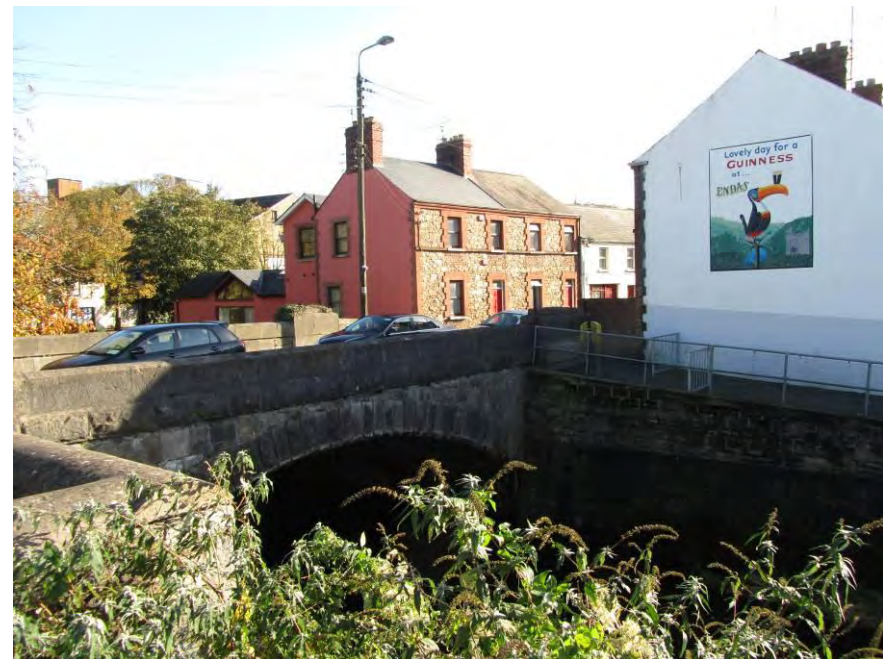
Fig. 59: Bridge seen from site of the former mill building
