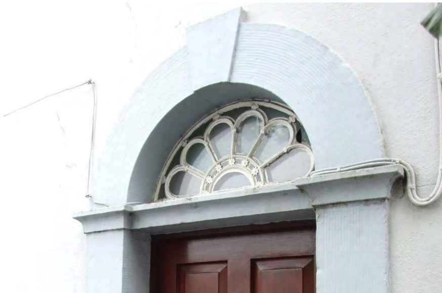
Fig. 116: Decorative fanlight on Irish Street
