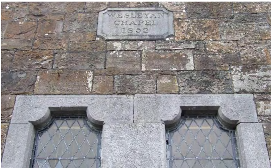
Fig. 109: Cut stonework to former Methodist Church
