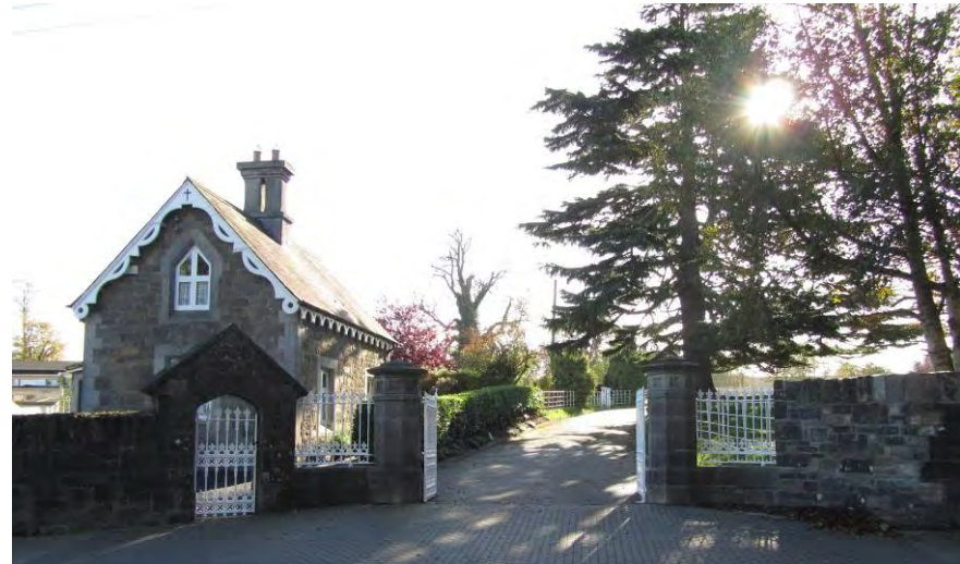
Fig. 89: Gate lodge and trees to the Convent of Mercy
