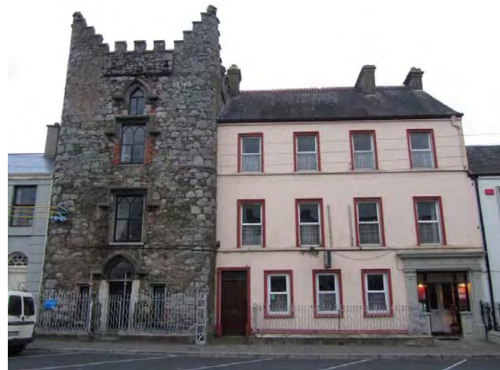
Fig. 51: Hatch's Castle, Market Street
