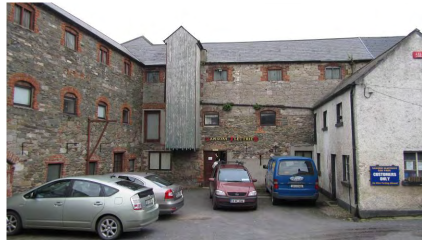
Fig. 61: Warehouses to rear of Ulster Bank, Market Street
