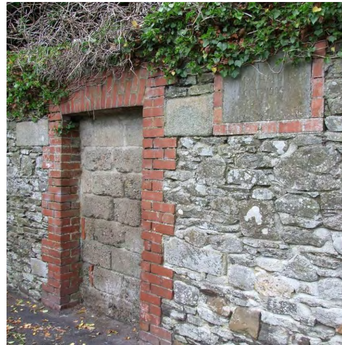
Fig. 70: Blocked doorway to rear of Hatch's Castle site
