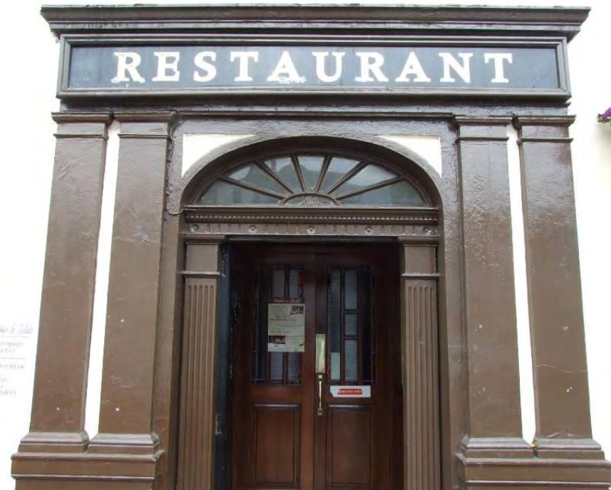
Fig. 55: Doorway on Castle Street
