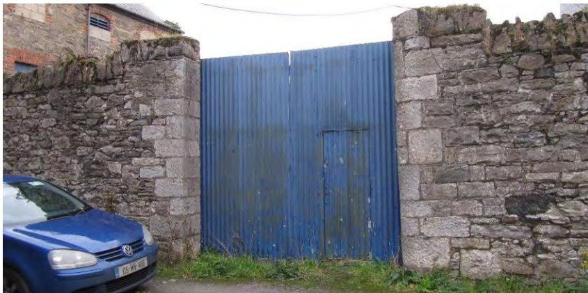
Fig. 60: Rubble stone wall with cut stone gate detailing
