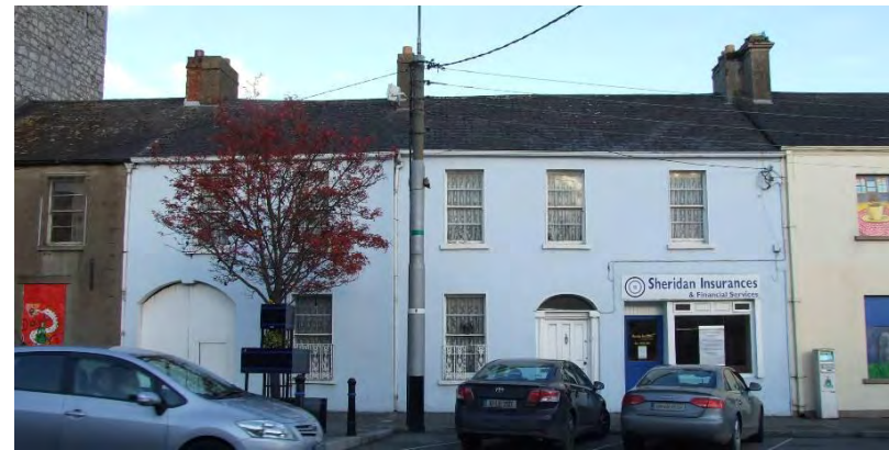
Fig. 24: Houses on east side of Castle Street
