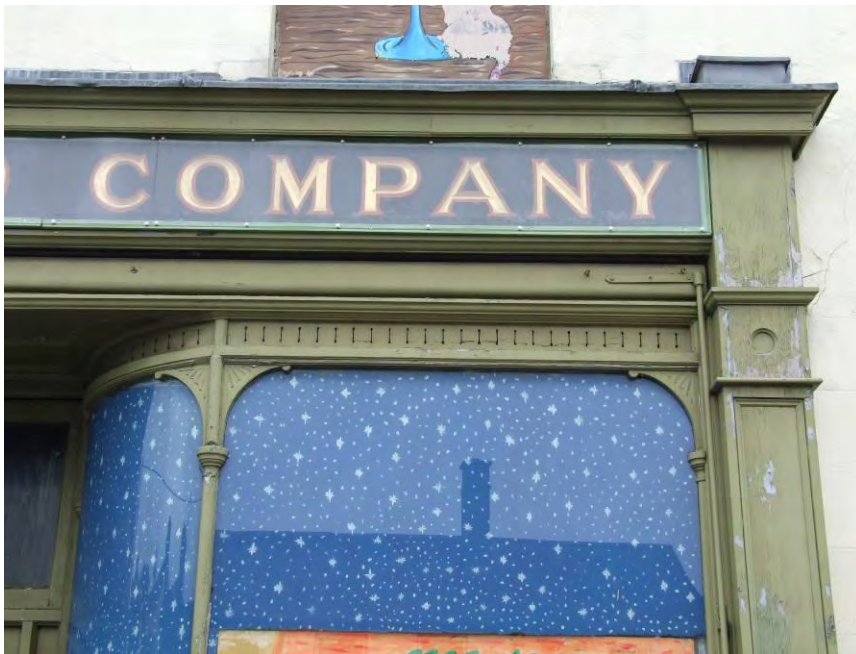
Fig. 25: Detail of shopfront on Castle Street
