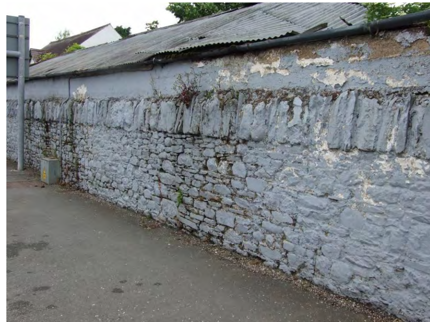
Fig. 104: Traditional stone masonry wall on Dundalk Road
