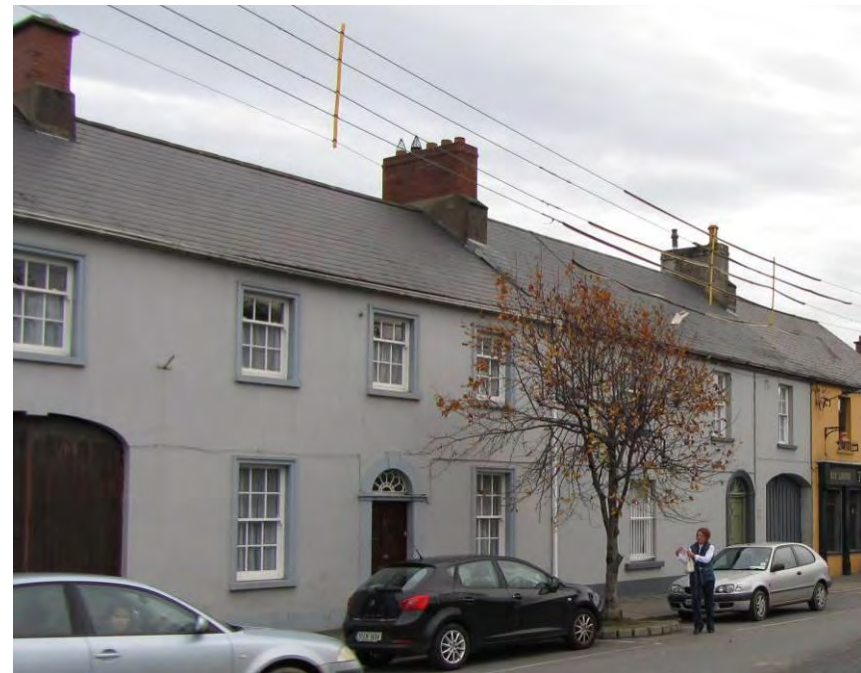
Fig. 23: Houses to east side of Irish Street
