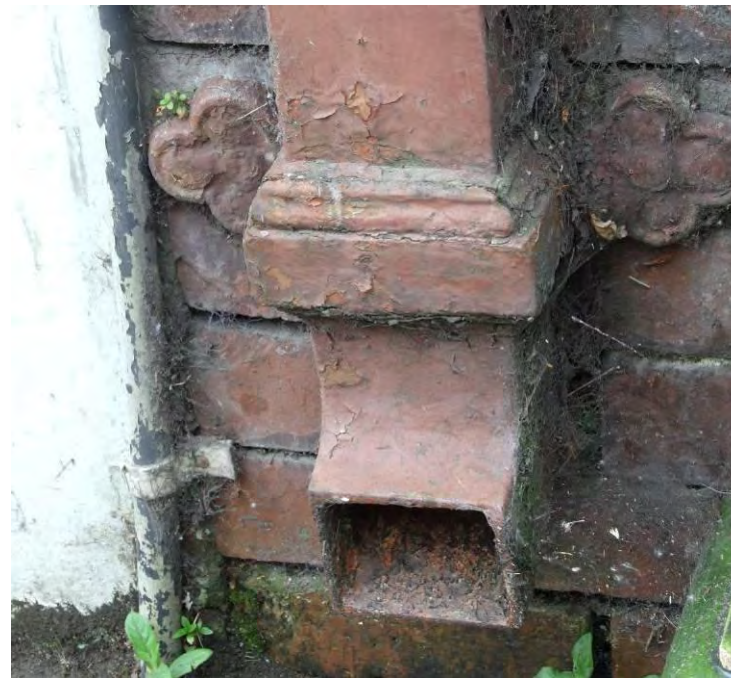
Fig. 108: Down pipe with decorative fixings, Bridge Street
