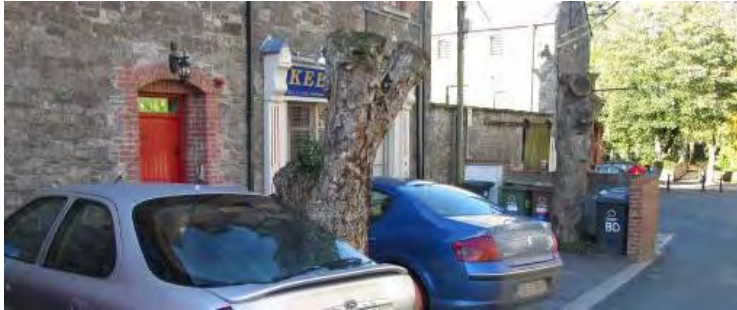
Fig. 136: Need for replacement trees and protection from vehicles
