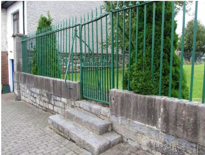
Fig. 46: Railings to St Mary's Church
