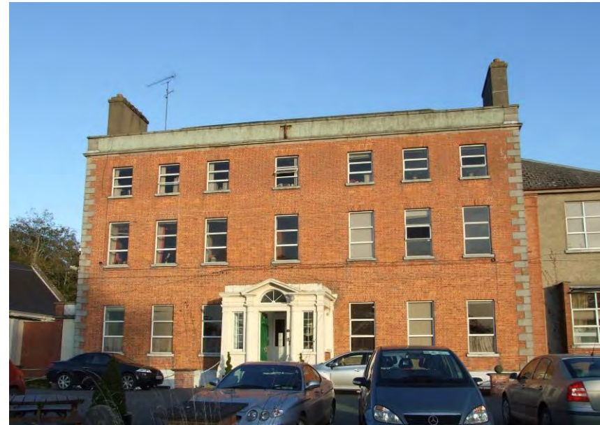
Fig. 93: View of the former Ardee House from the south
