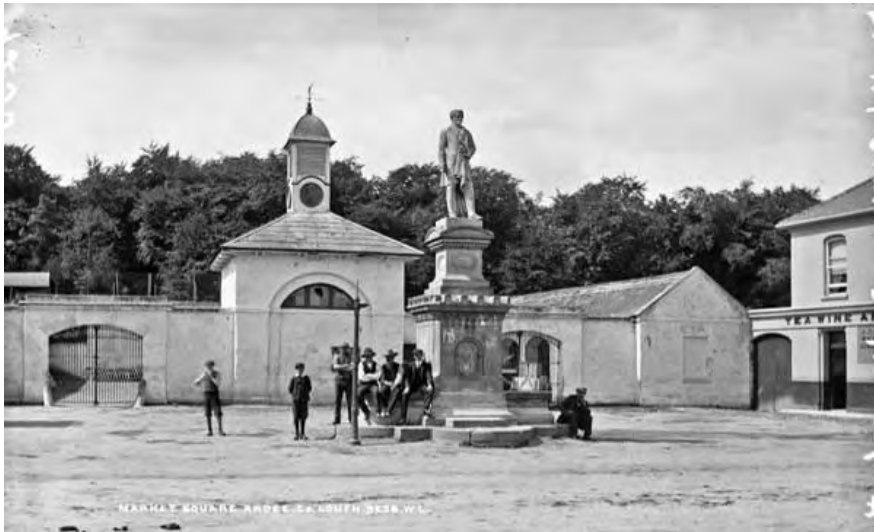
Fig. 14: Ardee market house and square, Lawrence Collection, c. 1900
