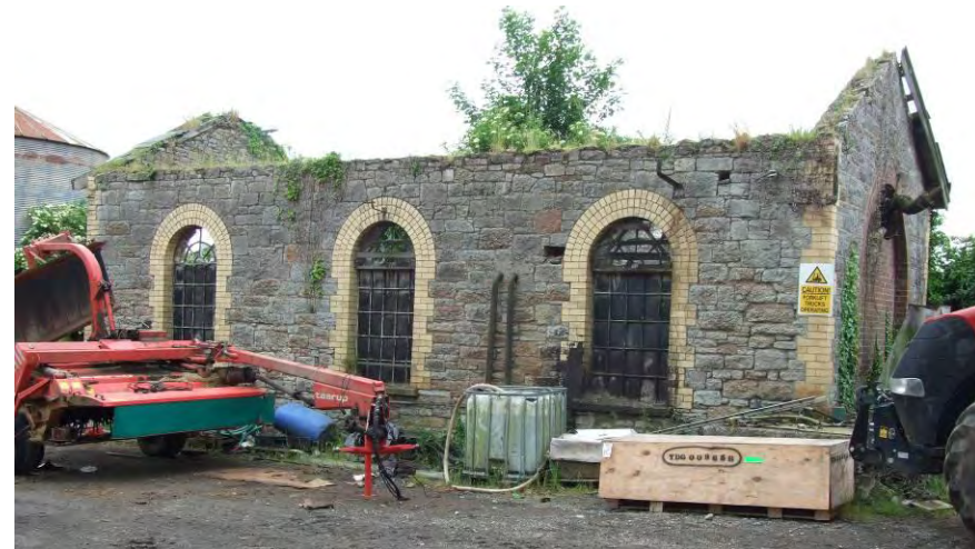
Fig. 67: Former station good shed
