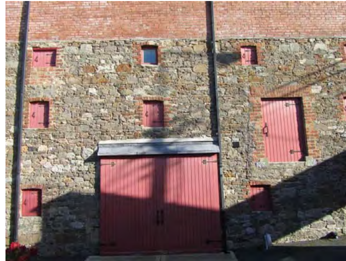
Fig. 112: Exposed brick and rubble stone wall
