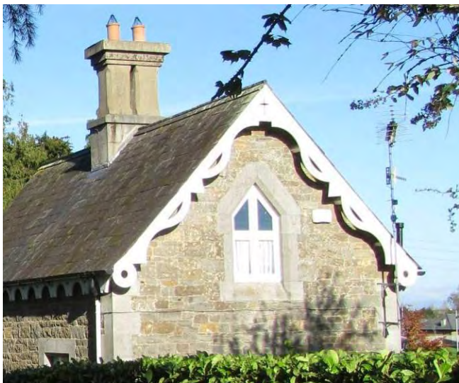
Fig. 107: Decorative bargeboards to convent gate lodge
