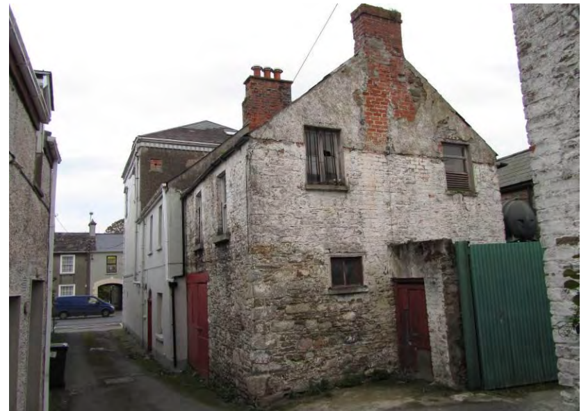
Fig. 62: Former dwelling to rear of Market Street
