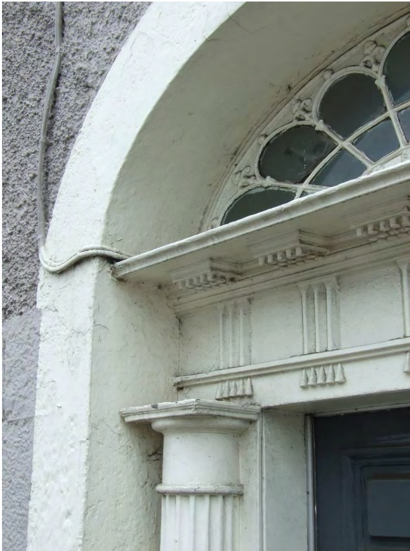
Fig. 103: Ionic detail to doorcase on William Street
