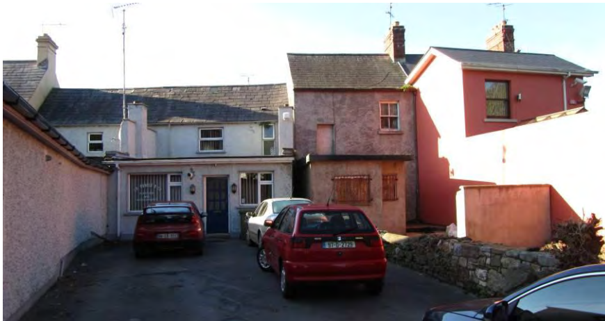
Fig. 133: Loss of rear boundary definition
