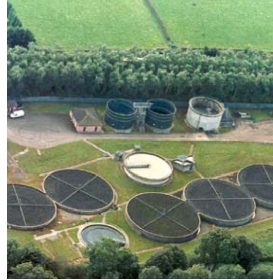
Ballyclare Wastewater Treatment Plant
