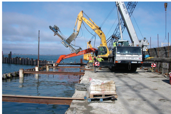
Works on upgrading and extension to harbour at Port Oriel
