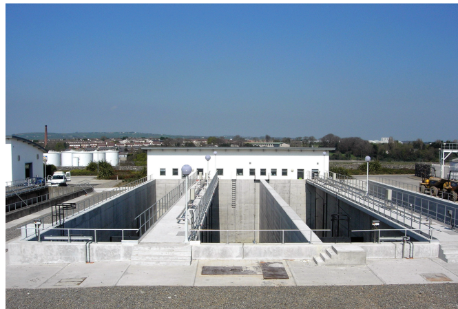
Extension to Drogheda Waste Water Treatment Plant.
