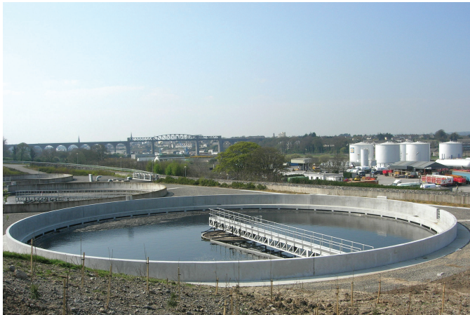
Drogheda Waste Water Treatment Plant.
