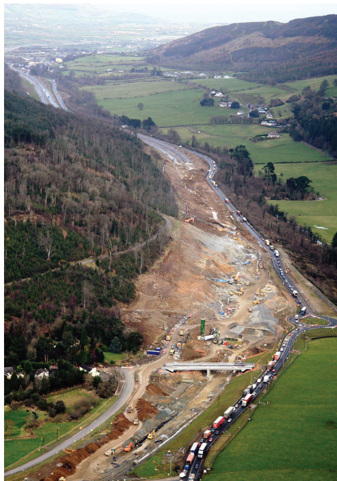
Aerial view of construction of the Newry-Dundalk Link Road.
