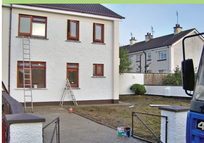
Before and after house refurbishment.
