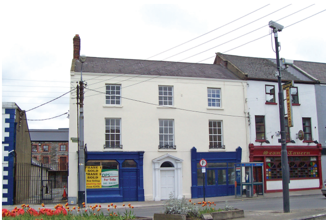
Shop front improvements under Town Renewal Scheme.
