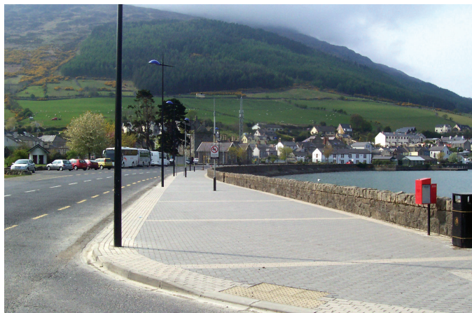
Paving and environmental improvements in Carlingford.
